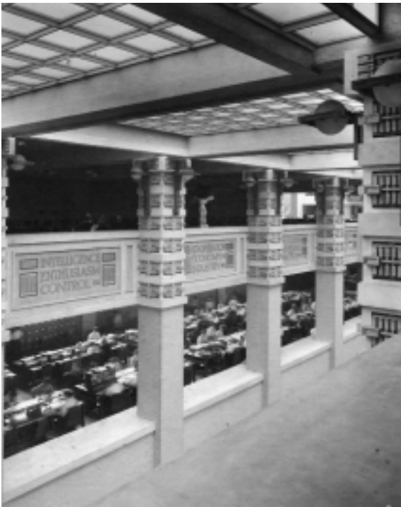
5 A masonry building with steel-framed interior. Larkin Administration Building, Buffalo. Frank Lloyd Wright, architect, Paul Mueller, builder, 1904–06, since demolished a Perspective from the Wasmuth folio, 1911 b Interior, showing steel beams (right-hand top)
