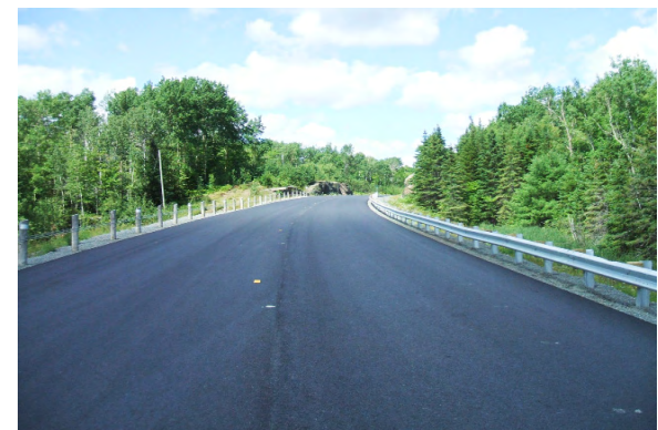
Completed Hwy 6 resurfacing
