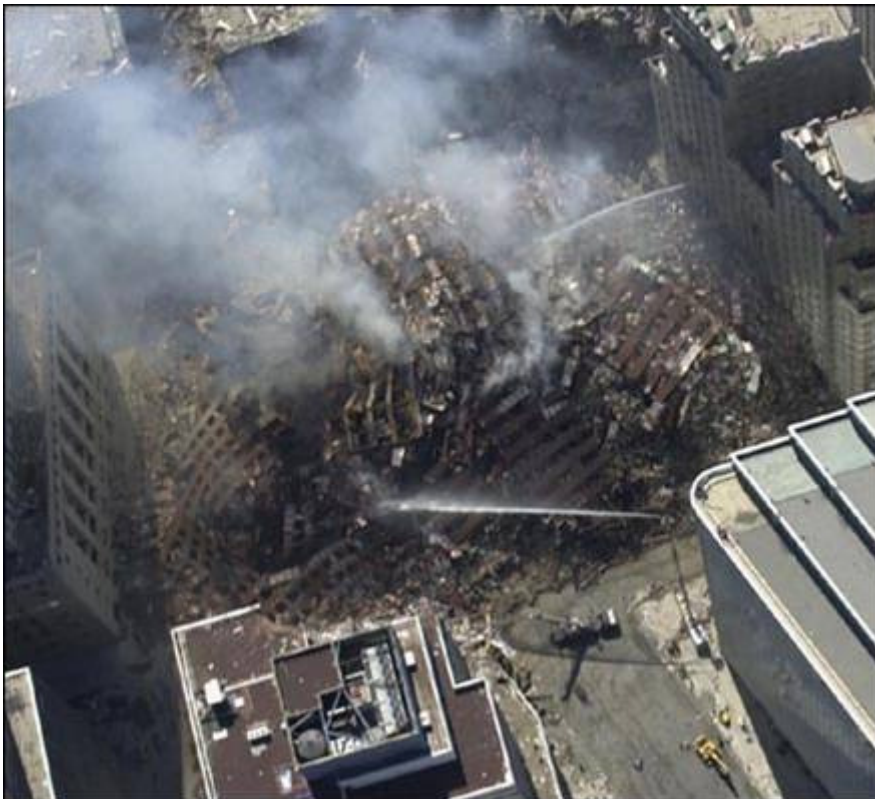
WTC 7 collapsed completely on 9/11/2001, primarily onto its own footprint.
