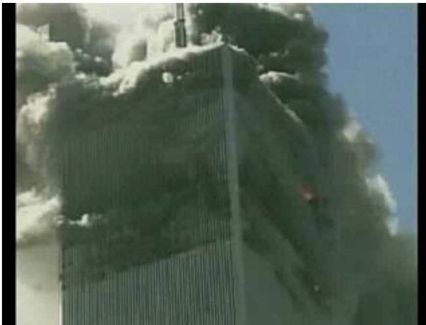
North Tower showing antenna (top) at beginning of collapse.
