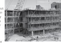
a three month delay and a \$3 million cost to remediate the soil, the Construction Schedule has proceeded as planned, with every major milestone being achieved. Currently, concrete is being poured to establish the four levels of the addition for the north half of the building addition, with basement utilities and under drain system installation ongoing for the south half of the building addition.
