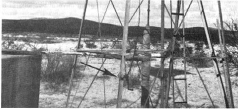
Windmill. Note windlass (arrow).
