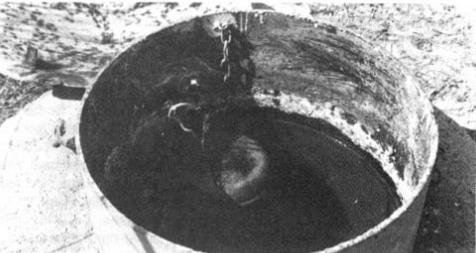
Float-valve regulates water level in stock tank.
