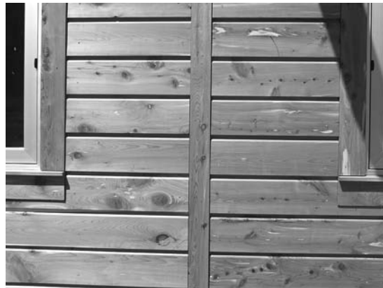
FIGURE 37. Finish Product in Place.
