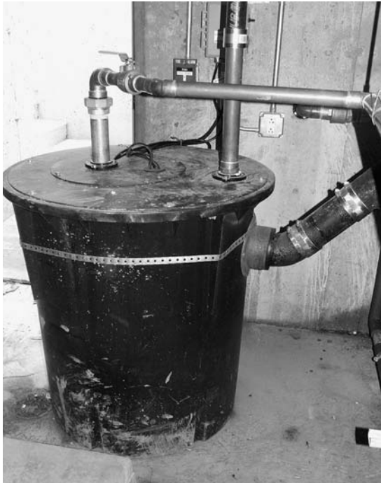
FIGURE 11. Nutrient Staging—Greywater Dosing Basin.
