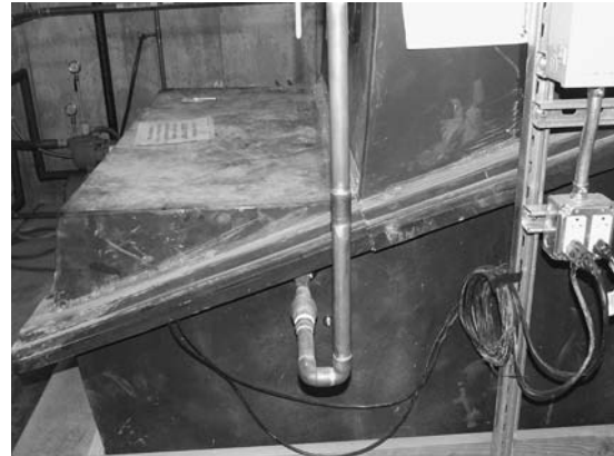
FIGURE 9. Compost Toilet—Misting System.
