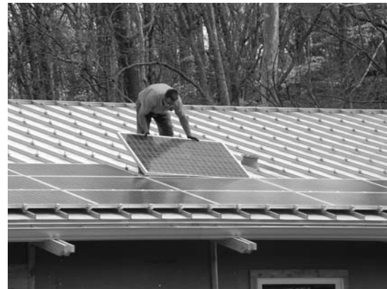
FIGURE 28. PV Panel Installation.
