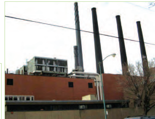
Power Plant—West Campus
