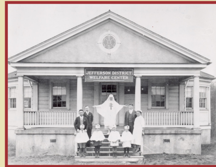
Alexandria County (which became renamed Arlington County the next year) established a Health Department in 1919 and constructed one of its clinics in Potomac in 1923 at 2704 Mount Vernon Avenue. The clinic was open one or two days a week, concentrating on pregnancy and infant care, functions later taken over by City agencies after town annexation. Seen here are most of the professional employees of the Arlington Health Department in December 1929: Director Peyton Chickester, MD, second from left; Sanitary Inspector Norbert Melnick, second from right; and Norma Davies, RN, a nurse shared with the school system, far right. Missing is infant nurse Minnie Rudasill, RN. On the far left is Henry Latane, MD, who gave tuberculosis tests as needed, and in the center is Sue Brown, RN, who organized the "Health Crusaders" in Mount Vernon School on a volunteer basis to teach the virtues of cleanliness and a healthy lifestyle to local children. The building was also used sometimes by the one-person County Welfare Department, which concentrated mostly on child abandonment and truancy cases, and by the county school system's full-time dentist.
