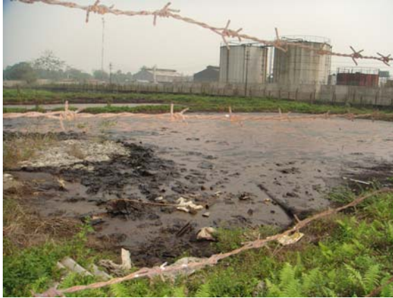
Earthen pits of crude / oily sludge inside Kathalguri mud preparation station
