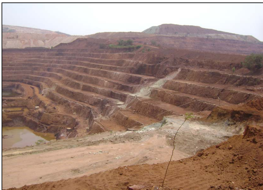
Typical Chromite Ore Mine Pit with Benches and Seepage Water collection
