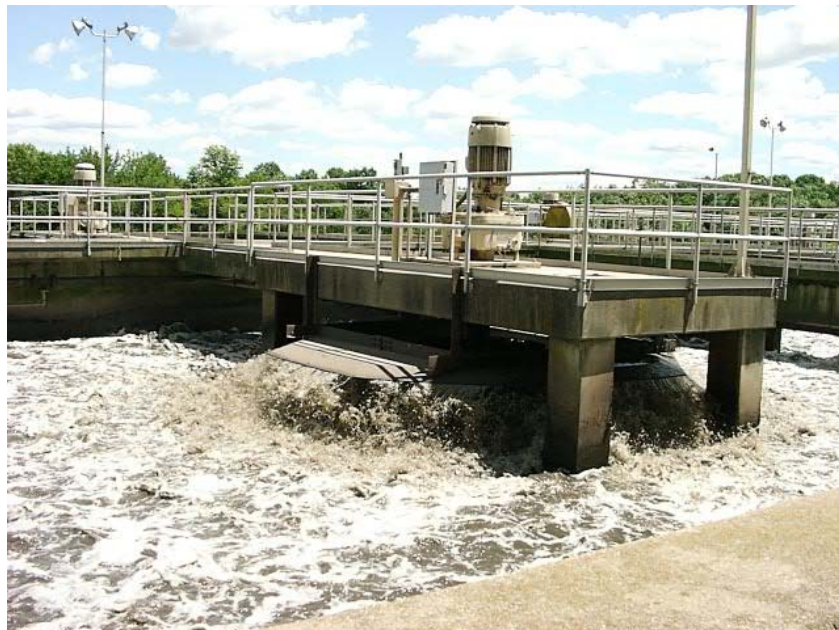
Effluent Treatment Plant
