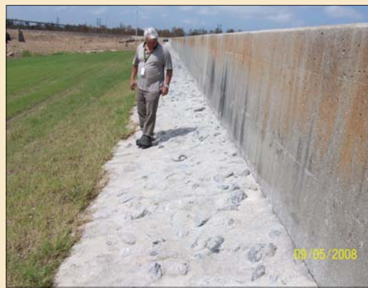
Assessment teams inspect areas after Hurricane Gustav
