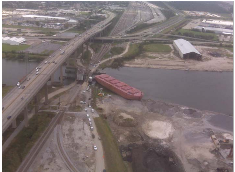
During Hurricane Gustav, more than a dozen unmoored vessels jammed this area, the railroad bridge just underneath the I-10 high rise at the IHNC.
