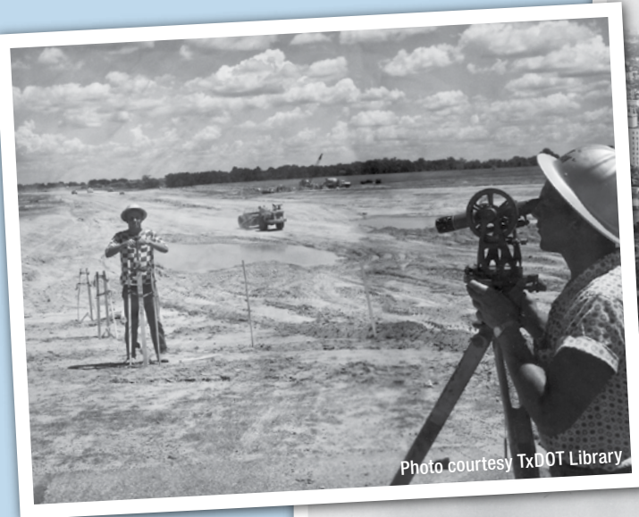
(Top): Construction workers survey land during an earth moving project on I-45 near Madisonville.
