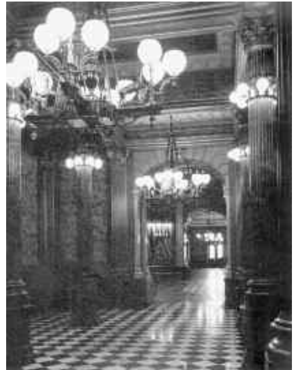
The entrance corridor on the first floor conveys the original elegance and craftsmanship of the Capitol. Restoration of the main corridors throughout the building involved stabilizing plaster; restoring decorative paint, including wood grained and marbled wainscot and wood-grained doors, doorframes and windows; restoring and improving lighting; restoring original marble and limestone tile floors; and installing an improved signage system.
