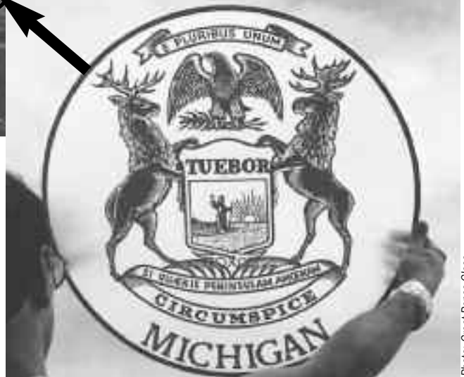
The coffered ceilings in both the House and Senate Chambers have been restored. Original panes of ruby-and-white hand-etched glass were lost years ago, replaced in the House by plastic and in the Senate by plywood. Replicas now feature the coats of arms of all 50 states, as well as Victorian designs and Michigan themes. A detail (right) shows Michigan's coat of arms. Skylights in the roof above let natural light into the chambers through these panels of glass.
