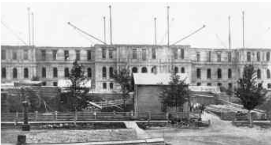
The Capitol under construction in 1875. Derricks rise above the walls, which have been completed to the second story.
