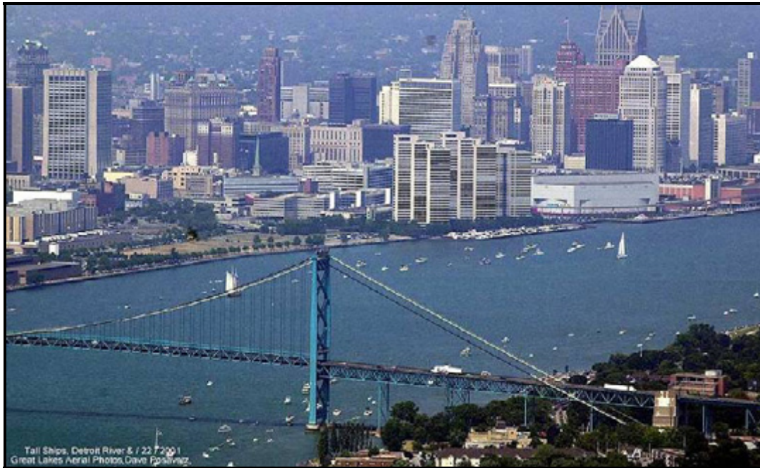
Figure 1 - Current Ambassador Bridge
