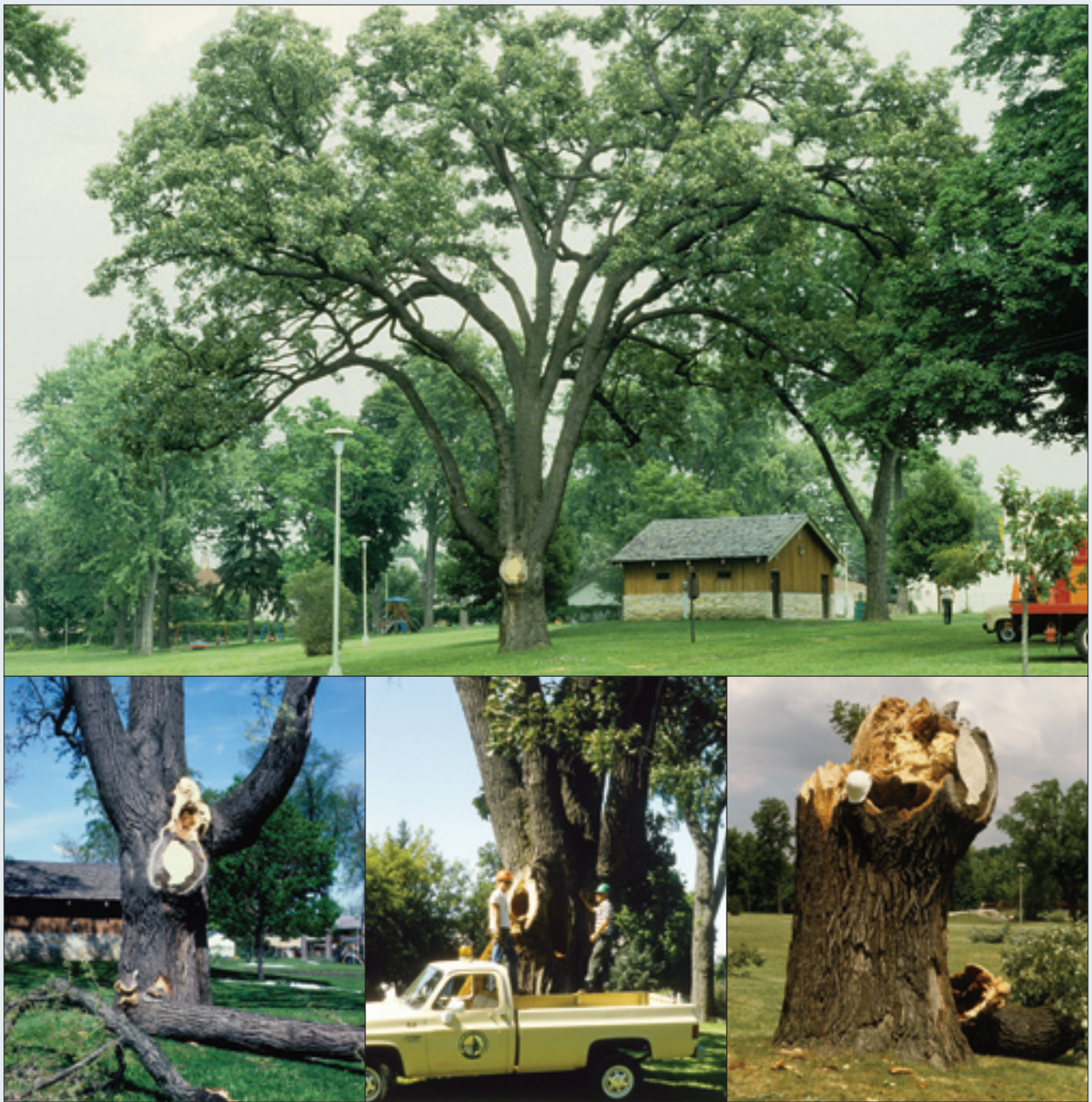
Figure 7. Extensive pockets of decay were exposed when this historic bur oak lost a lower scaffold limb. Cavity treatments and the cabling of the remaining lower scaffold limbs prolonged the life of the tree. The defect persisted, despite treatment efforts, and complete trunk failure occurred seven years after treatment at the point of decay.
