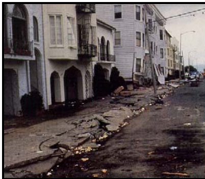
Liquefaction damage, Marina District, 1989 Loma Prieta, California, Earthquake Source – M. Bennett, U.S. Geological Survey
