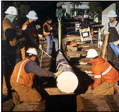
Gas pipelines being replaced in San Francisco
