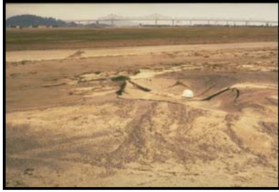
1989 Loma Prieta Earthquake - Alameda Naval Air Station
