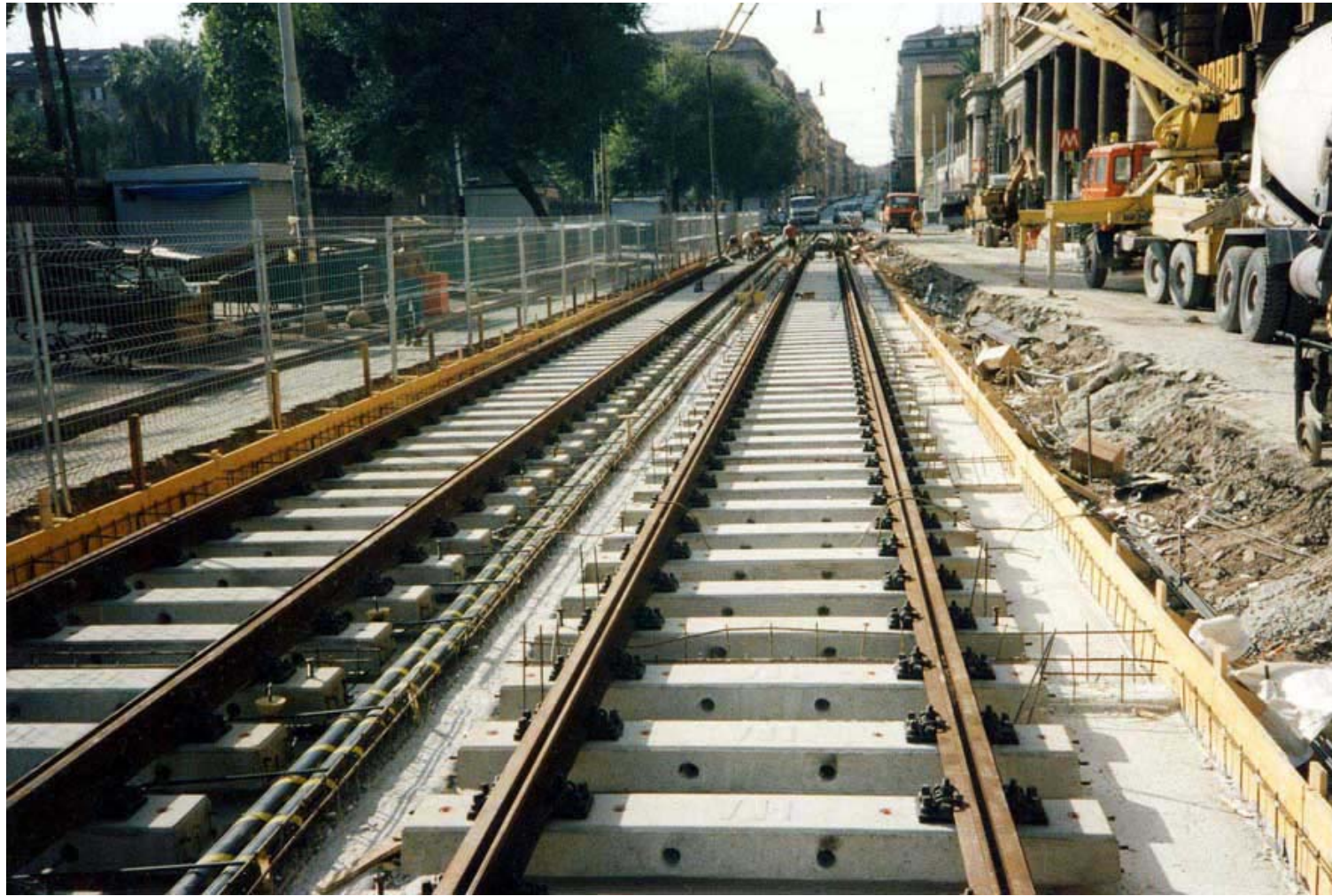
FIGURE 7 Piazza Vittorio Emanuele under construction.
