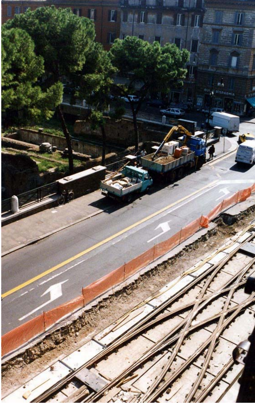
FIGURE 10 Piazza di Torre Argentina: tracks have been laid upon the precast concrete platform near Roman monuments dating back to the 3rd century B.C.
