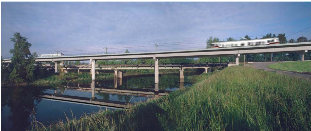
FIGURE 5 LRT structure (near side) higher than the highway structure (far side).
