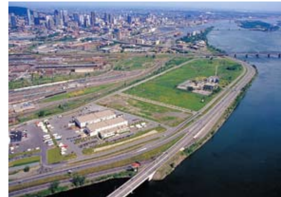
The same construction methods which extended Ile Ste Hélène and created Ile Notre Dame might be used to extend the shoreline of Pointe St. Charles. Source: Société du Havre
