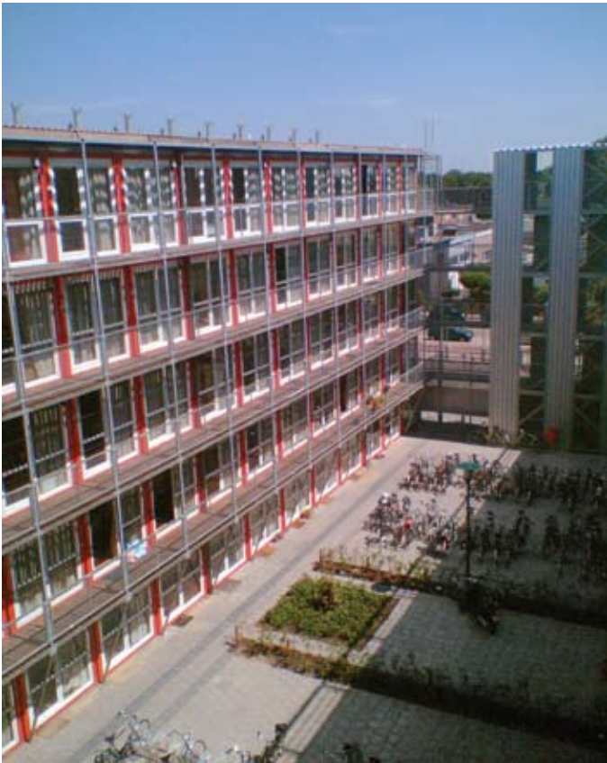
The recently completed Keetwonen housing project in Amsterdam comprises 1000 living units as well as a supermarket, office buildings and a restaurant. The entire complex was assembled with ISO dry freight containers. Source: TEMPOHOUSING
