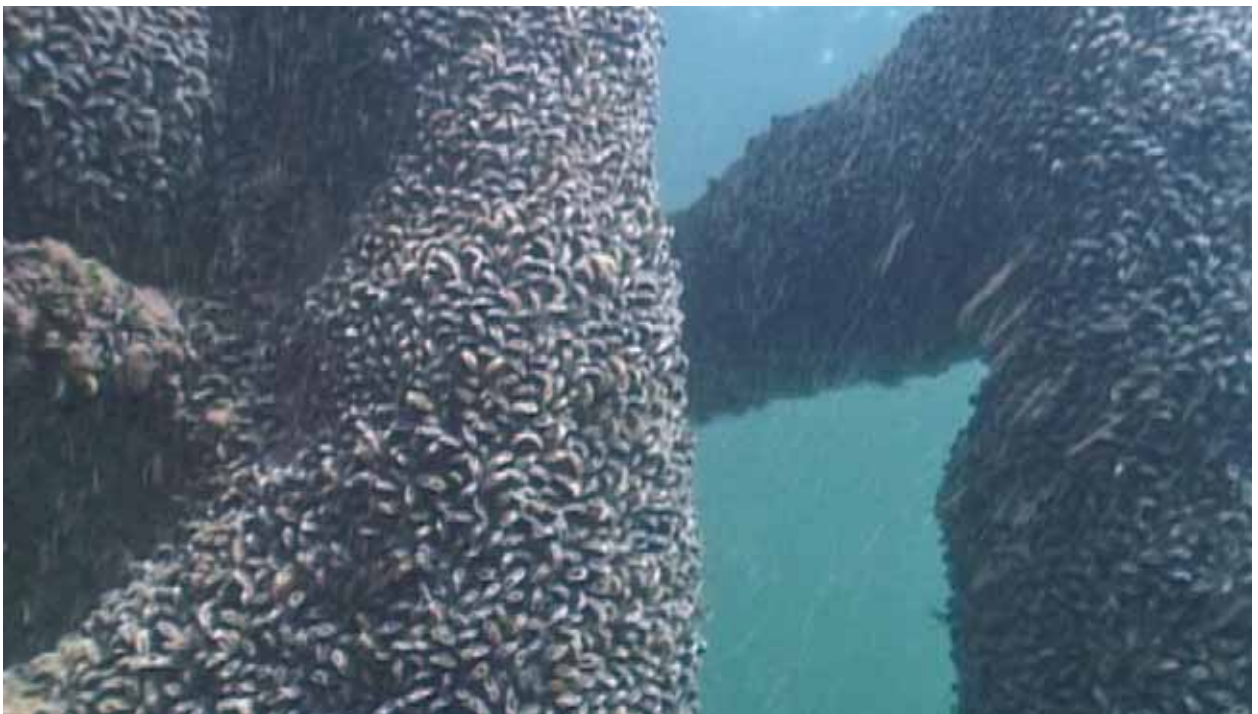
FIGURE 4.12 Common mussel on turbine structures at Horns Rev.
