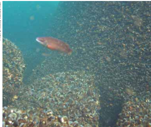
FIGURE 1.5 Scour protection with common mussels at Nysted.
