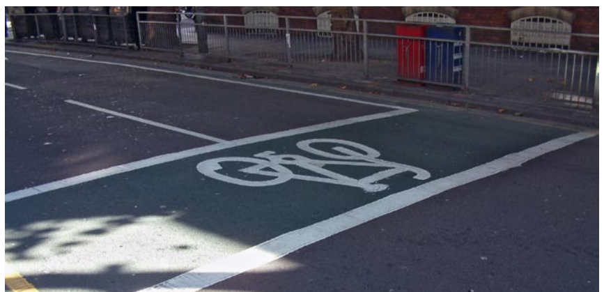
Fig. 9.23 and 9.24 In Chinese cities such as Xi'an (upper left photo) cyclists are given designated waiting areas from which they have priority access to crossing the street. Likewise, in the UK (lower photo), a priority bicycle stopping area is placed ahead of the stopping line for motorised vehicles.
