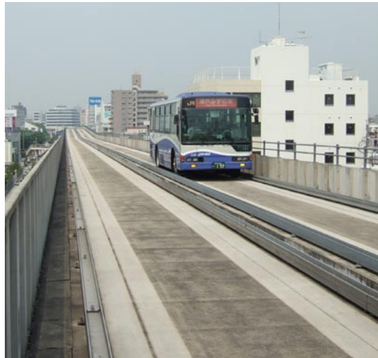
Fig. 5.30 The Yutorito line in Nagoya utilises an elevated roadway structure to avoid any conflicts with street level traffic. Photo by Lloyd Wright
