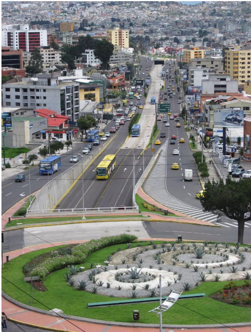
Fig. 9.54 Quito’s Central Norte line uses a series of underpasses to avoid a roundabout near Plaza Américas.
