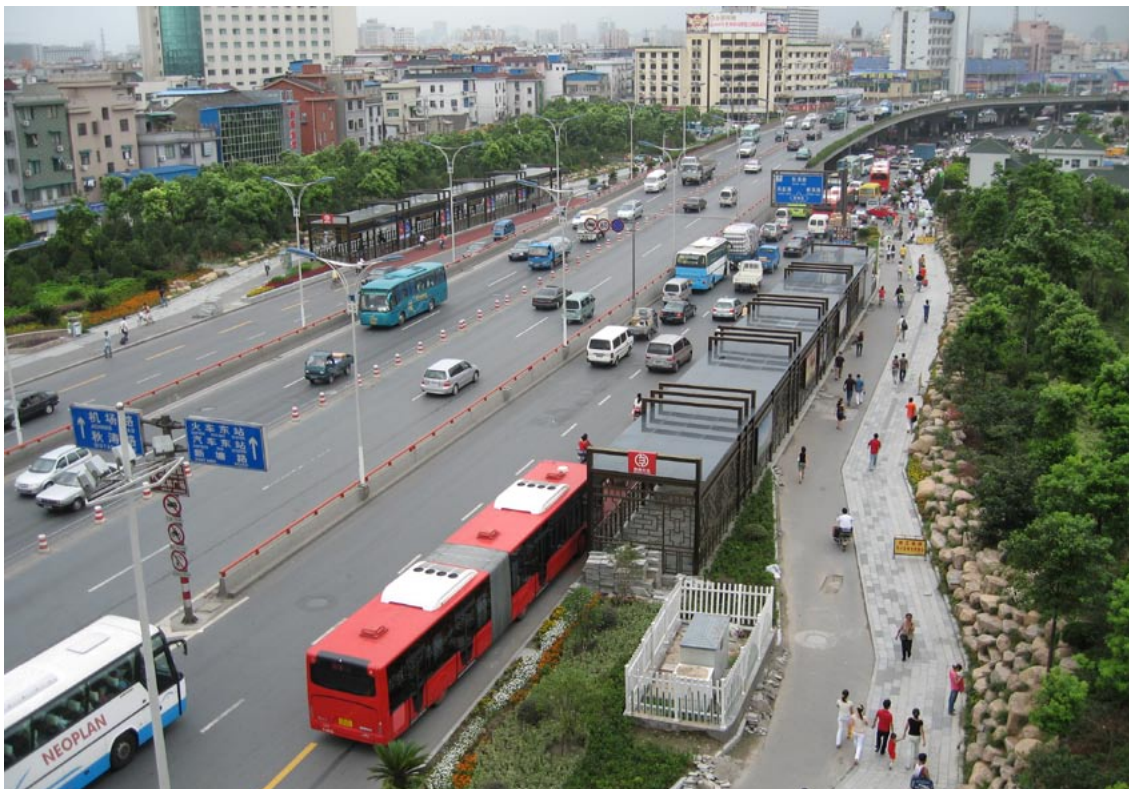
Fig. 13.102 The cycleway along the Hangzhou BRT system is sited between the BRT lane and the pedestrian footpath.
