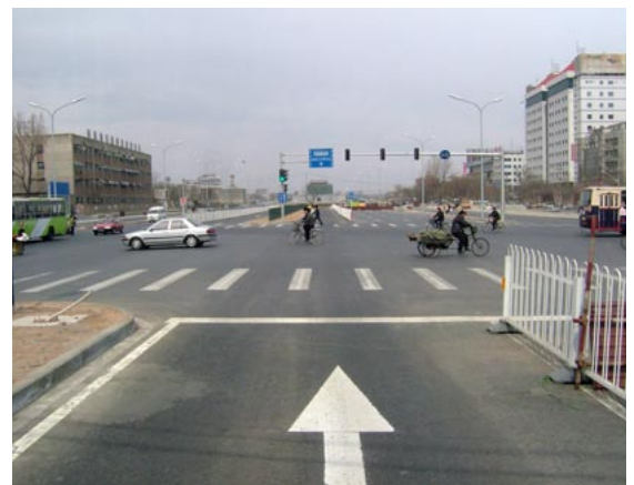
Fig. 3.26 The five-metre wide corridor in Beijing was quite wide for a single lane busway but insufficient for two lane operation.
