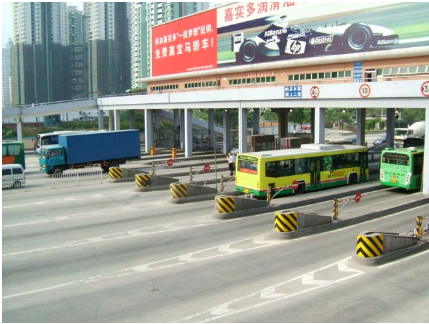
Fig. 13.35 Authors successfully testing an abandoned toll plaza on a high speed road in Guangzhou as a possible safe pedestrian crossing for a very wide high speed road.
