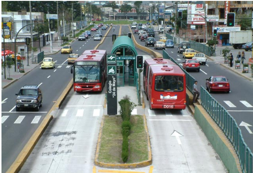
Fig. 5.6 The Ecovía corridor in Quito provides an example of a standard BRT road configuration. Photo by Lloyd Wright
