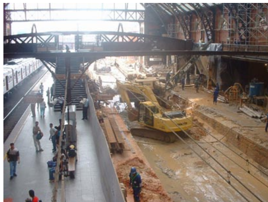
Fig. 2.27 and 2.28 An initial BRT corridor may take 12 to 24 months to construct (left photo); by comparison a typical underground or elevated rail system will require from three to ten years (right photo).
