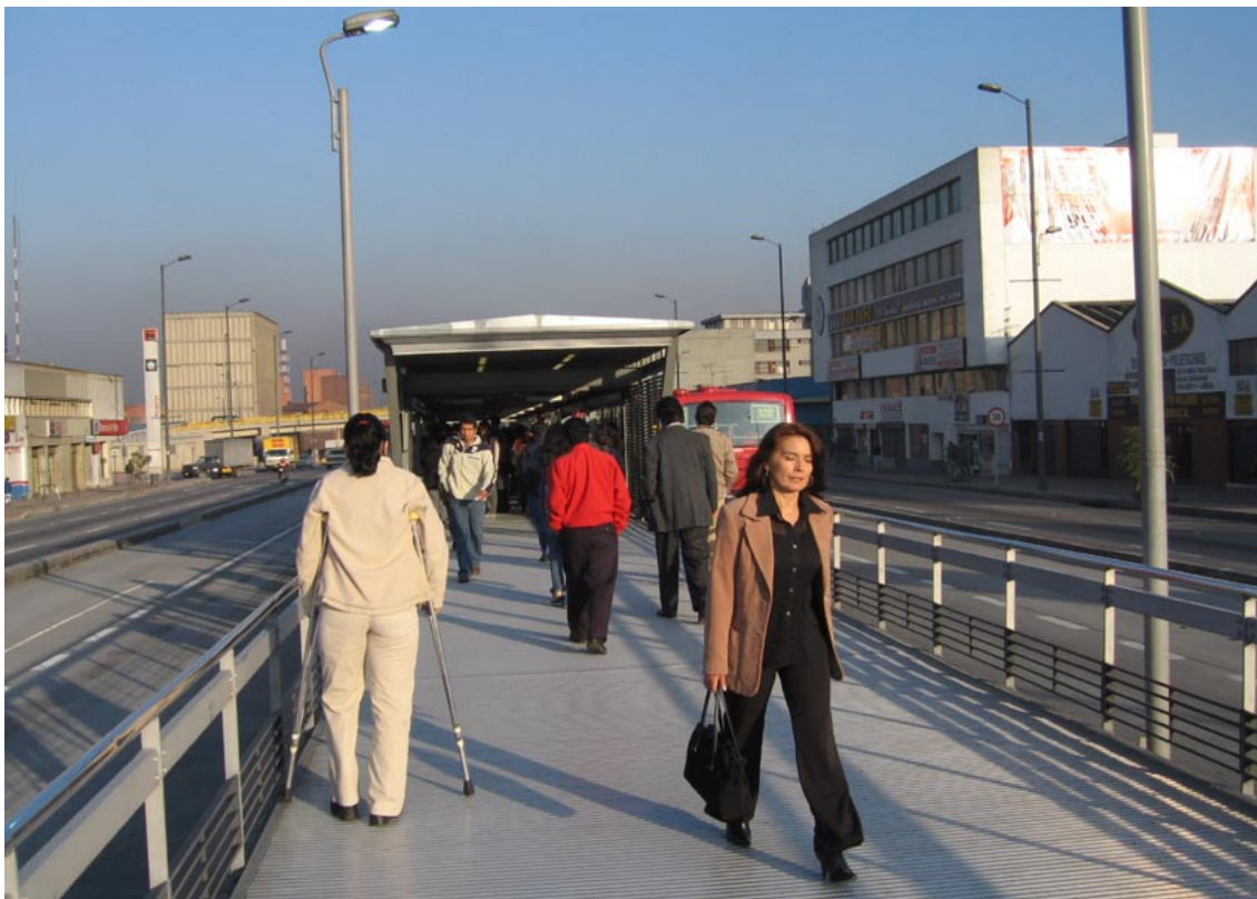
Fig. 13.72 The level station floors and platform transfers in Bogotá make it easy for anyone to move from one route to another.
