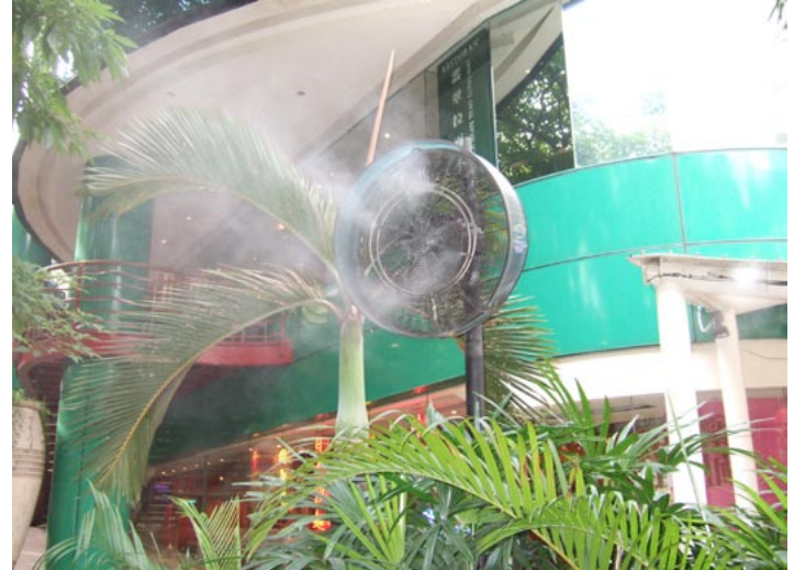
Fig. 11.56 and 11.57 Mist generators and ventilator fans are a cost-effective alternative to air conditioning as shown in these examples from the Pattaya (Thailand) bus terminal (left photo) and along a street in Kuala Lumpur (right photo).
