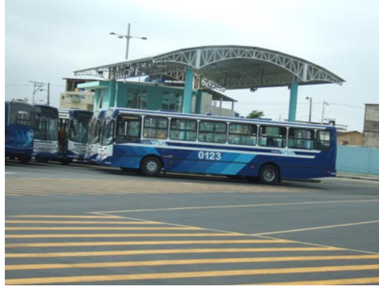
Fig. 11.120 and 11.121 The architecture for the maintenance areas in both Bogotá (left photo) and Guayaquil (right photo) is both aesthetically pleasing and highly functional. Photos by Lloyd Wright
