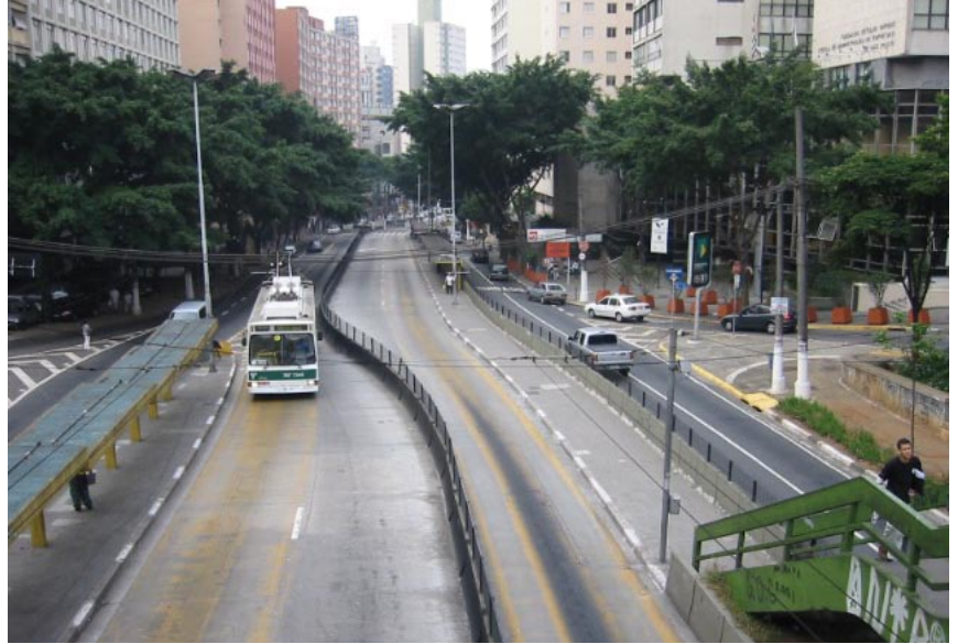
Fig. 11.16 Prior to its removal, the wall barriers on the São Paulo Novo de Julio corridor undermined the urbanistic qualities of the corridor.
