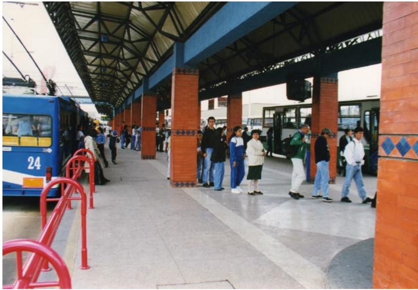
Fig. 11.93 At the El Recreo terminal of the Quito Trolé, customers easily transfer from trunk services to feeder services by crossing a platform.
