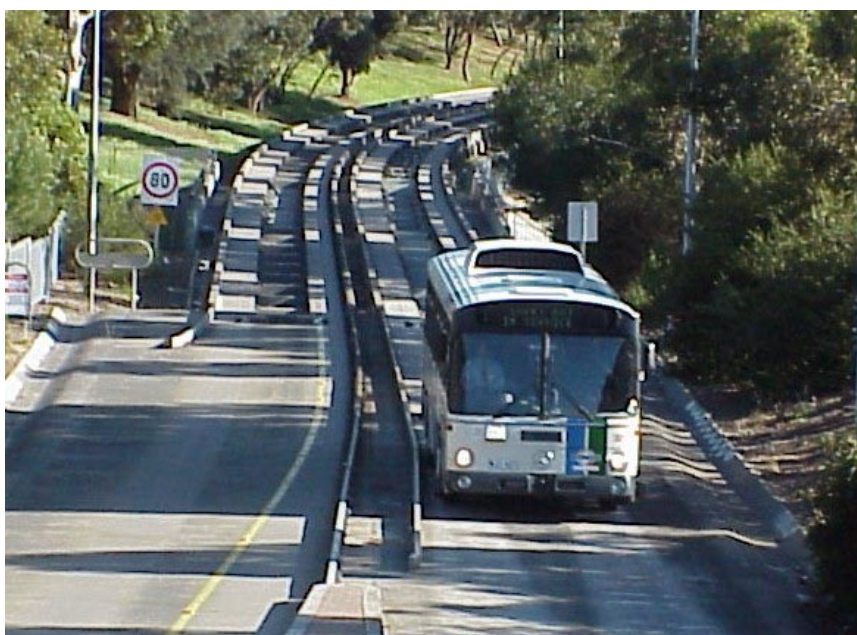
Fig. 11.24 Mechanically guided systems allow greater vehicle velocities and narrower busway width, but these systems tend to increase construction costs and reduce overall system flexibility.
