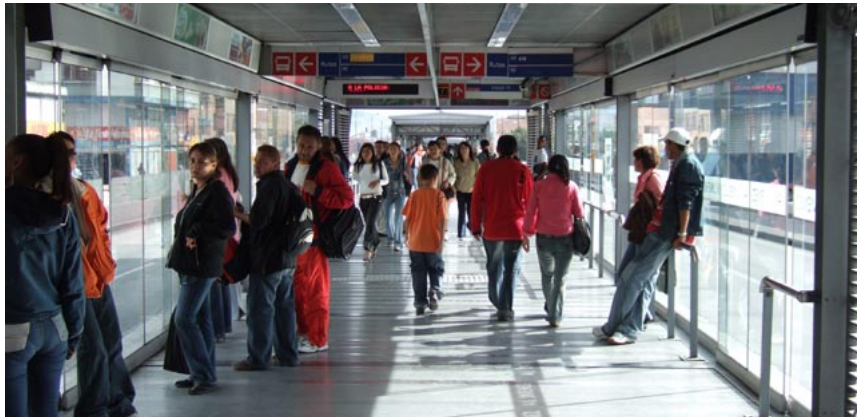
Fig. 11.87 Bogotá utilises stations with multiple stopping bays in order to permit platform transfers for customers wishing to change from one route to another.
