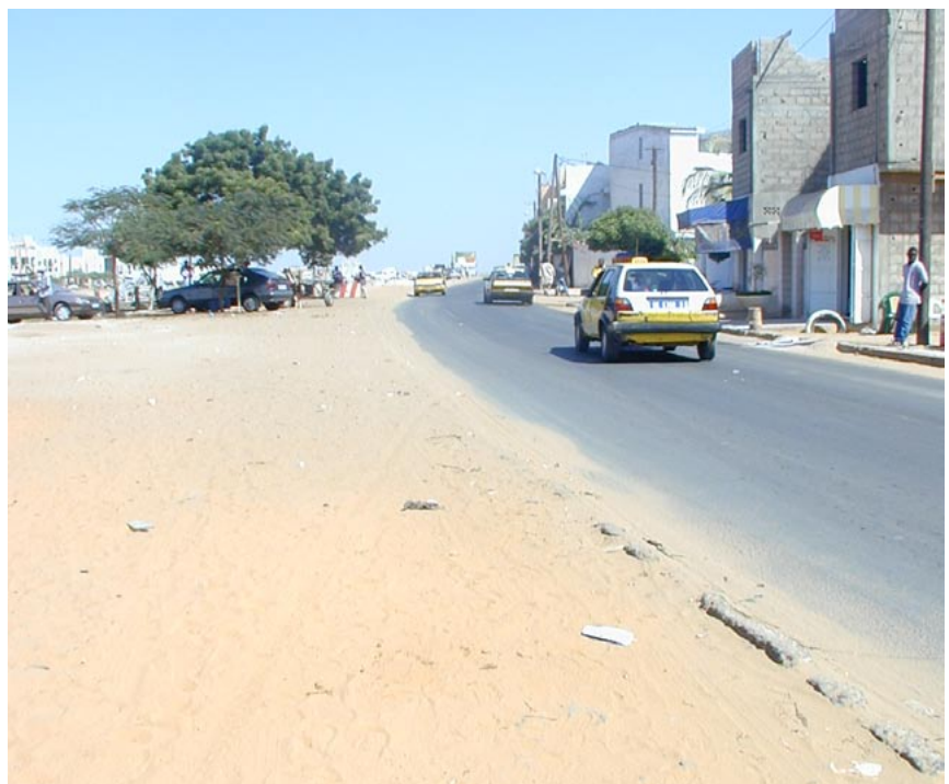
Fig. 5.21 The VDN corridor in Dakar will likely make use of available right-of-way space in the median to construct the BRT lanes. Photo courtesy of ITDP
