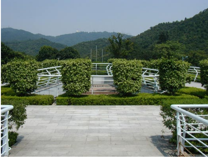
Fig. 13.53 A park-like environment makes this pedestrian overpass in Guangzhou (China) more inviting.
