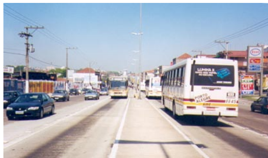
Fig. 8.40 and 8.41 Convoying allows the Porto Alegre system to achieve peak capacities of over 20,000 pphpd, but at the same time this technique can result in busway and station congestion and therefore slowing average vehicle speeds. Photos by Lloyd Wright
