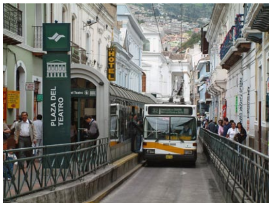
Fig. 5.13 The narrow right-of-way space and high passenger volumes at the Quito “Plaza del Teatro” station have necessitated the physical separation of the busway and the pedestrian space.
