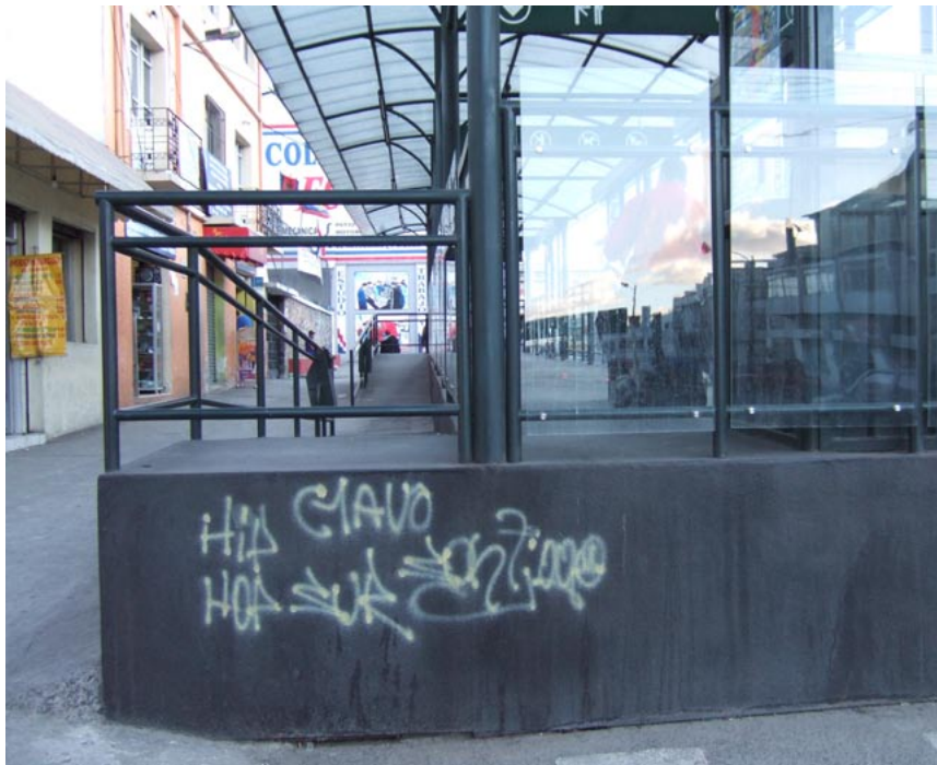
Fig. 17.49 Without a dedicated maintenance fund for dealing with problems such as graffiti, the quality of a system can quickly deteriorate.
