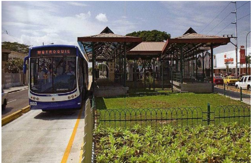
While the Curitiba tubes have been quite successful in creating an iconic image for the city, there are a few limitations to this type of design which could restrict its use elsewhere. First, the rounded design can be a limitation of system
