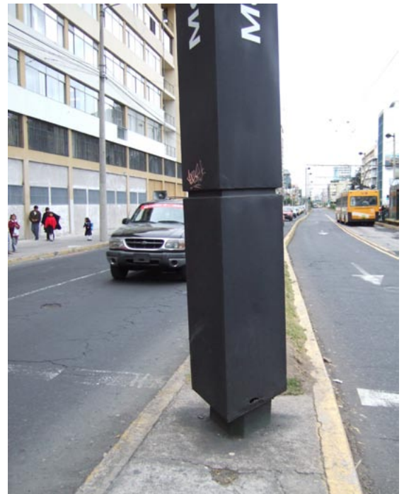
Fig. 13.61 This BRT identification post in Quito is placed in a pedestrian island, and acts to block the pedestrian’s view of both oncoming mixed traffic as well as oncoming BRT vehicles.
