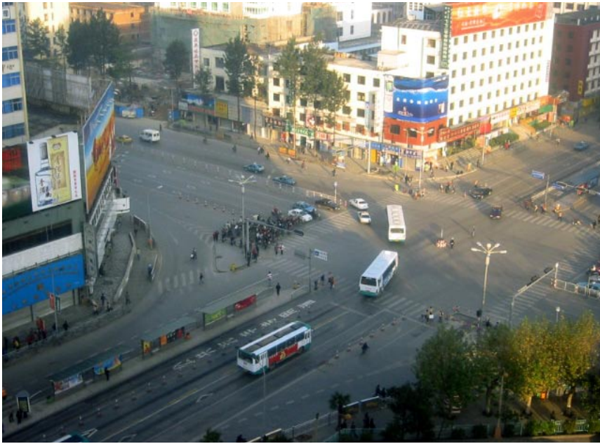
Fig. 9.35 In Kunming, turning BRT vehicles leave the busway and enter a mixed-traffic lane to finalise the turning movement.
