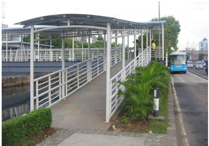
Fig. 13.25 The addition of higher-quality pedestrian crossings in Jakarta has done much to reduce pedestrian accidents.
