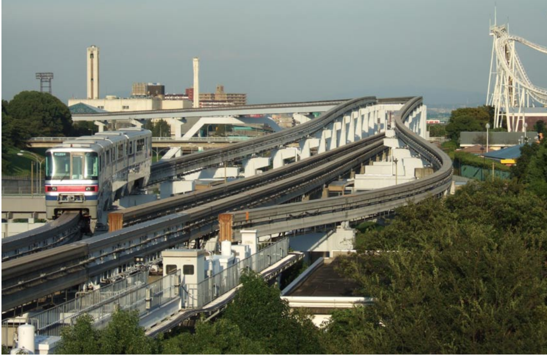
Fig. 2.43 As this image from the Osaka monorail indicates, in order for two intersecting rail corridors to cross in high-capacity urban conditions, grade separation is likely to be necessary.
