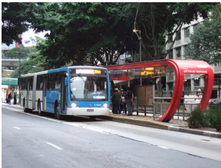
Fig. 5.63 São Paulo utilises buses with doorways on both sides of the vehicle in order to service both median and curbside stations.
