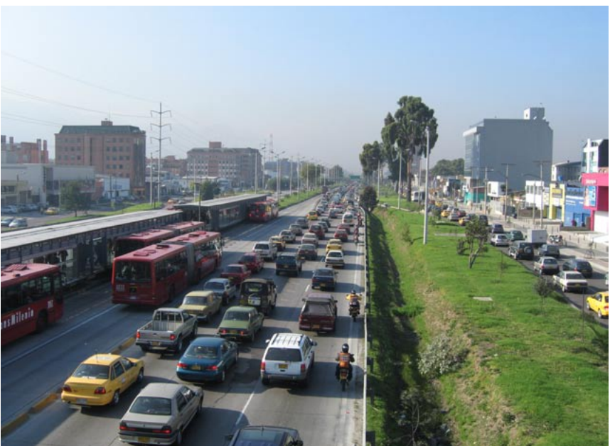
Fig. 8.36 The existence of a passing lane makes the high passenger capacities achieved in the Bogotá system possible.
