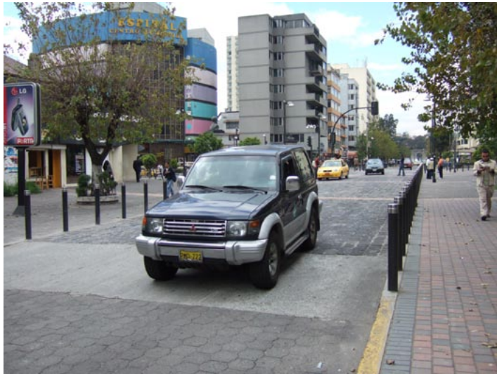
Fig. 13.29 Raised intersection in Quito.
