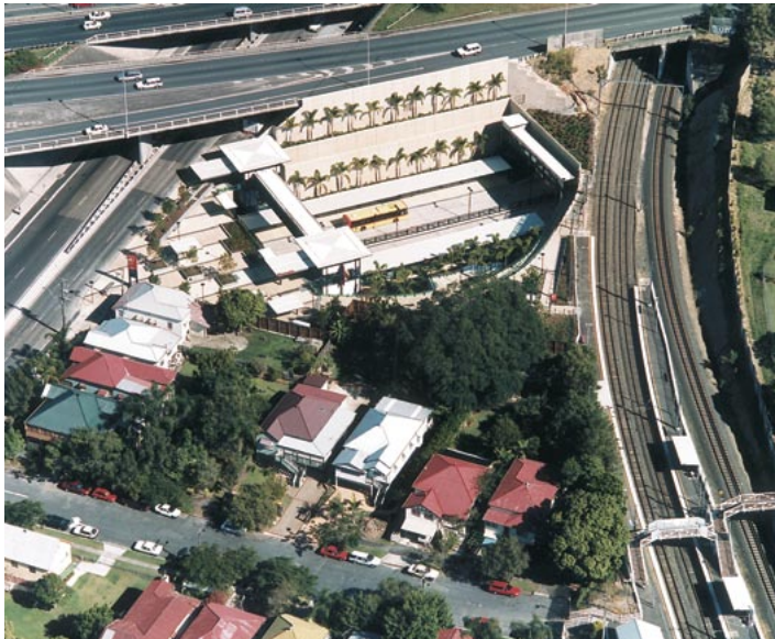
Fig. 13.108 The Brisbane Busway (top centre) is closely integrated with the city's commuter rail service (right).
