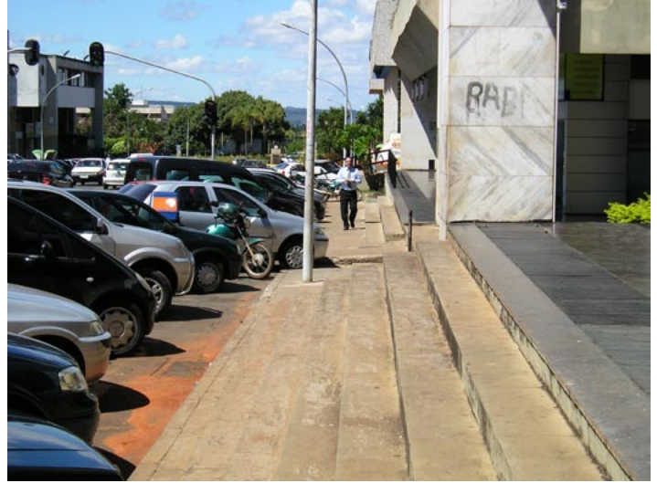
Fig. 13.66 These steps in Brasilia (Brazil) reduce the effective width of the footpath to less than 0.5 metres.
