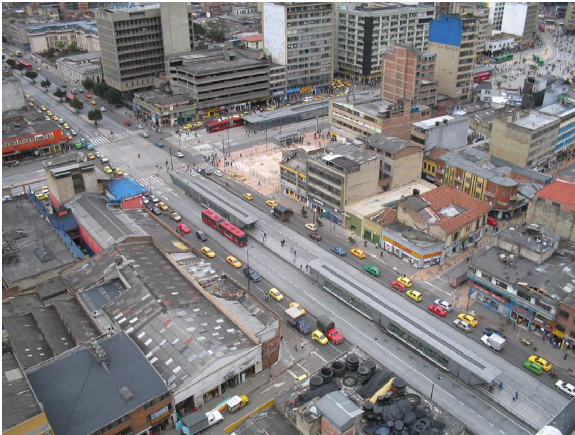
Fig. 8.5 The use of multiple stopping bays and passing lanes in Bogotá helps minimise bus congestion.
