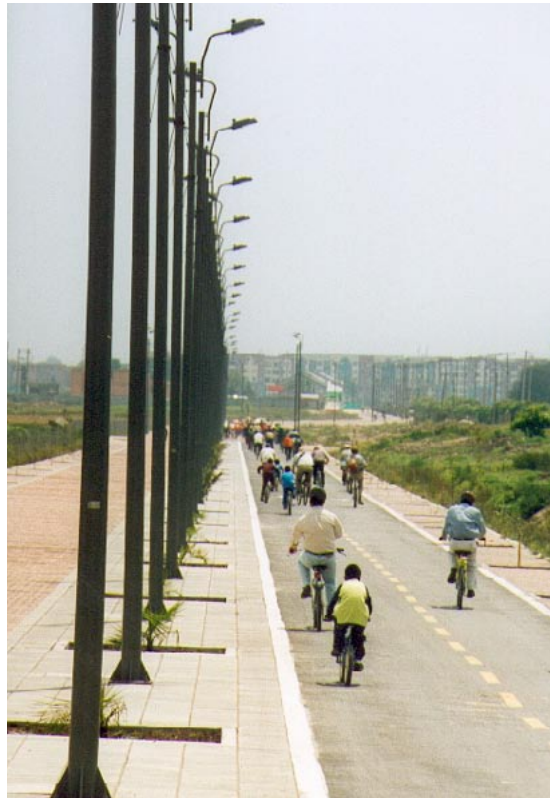
Fig. 19.37 High-quality pedestrian and cycleway facilities connect low-income communities with the TransMilenio system in Bogotá.
