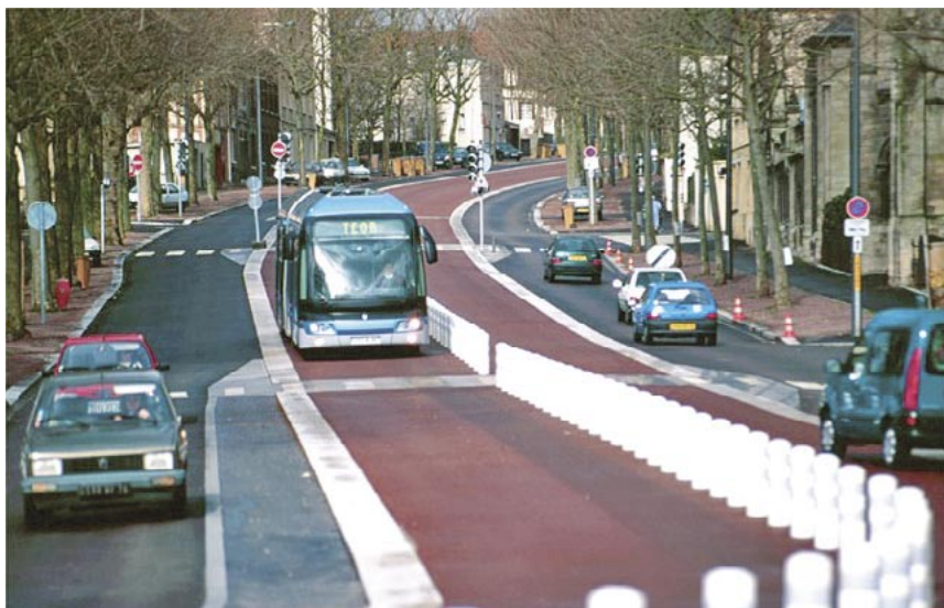
Fig. 5.7 BRT corridors can also function adequately with the provision of only a single lane of mixed traffic, as shown in this example from Rouen (France). Photo courtesy of TCRP photo library
