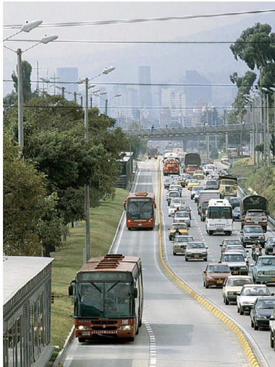
Fig. 7.29 and 7.30 Passing lanes at stations as practiced in Bogotá (left photo) and São Paulo (right photo) allow for the provision of express and limited stop services, which deliver significant travel time savings to customers.
