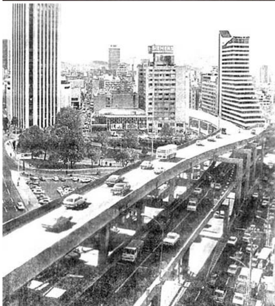
Fig. 3.12 A JICA drawing showing a vision for Bogotá with elevated roadways. Fortunately, Mayor Enrique Peñalosa rejected this vision and opted to build TransMilenio instead of elevated roads. Image courtesy of the Municipality of Bogotá
