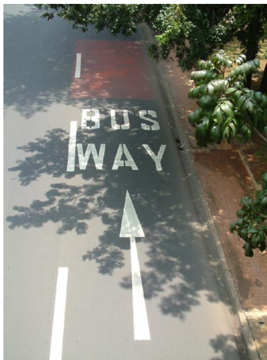
Fig. 11.33, 11.34, and 11.35 Signage is a basic mechanism to designate an exclusive busway, as seen in these examples from León (top photo) and Jakarta (middle photo). Painted information on the busway surface is also an option, as show here form the example in Jakarta (bottom photo).
