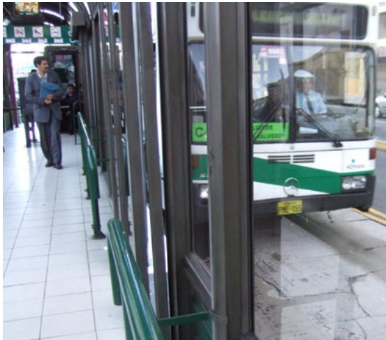
Fig. 10.5 With no announcements or electronic display, customers on the Quito Trolé only have a brief, sight-line impaired view of the route number for the vehicle approaching the station.
