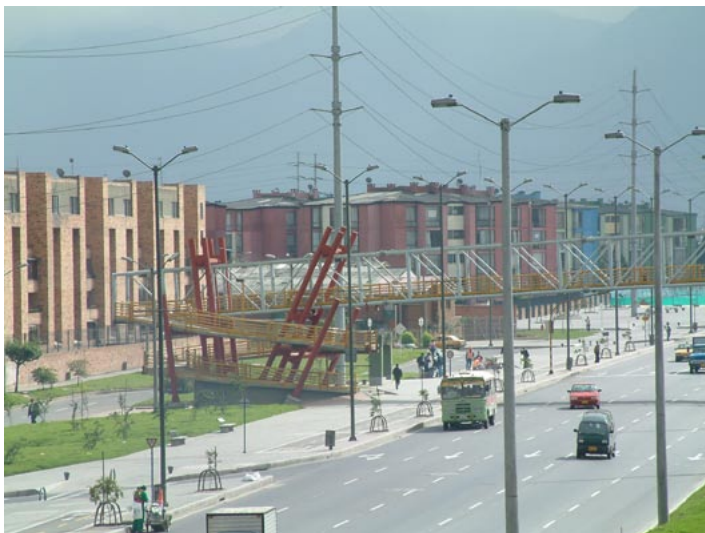
Fig. 13.48 In conditions where the BRT station is in the median of a multi-lane expressway, Bogotá utilises a pedestrian overpass.
