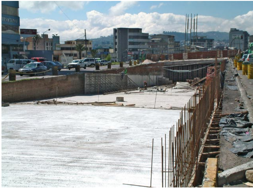
Fig. 20.32 Re-routing traffic around intersections that are under heavy construction can be particularly challenging.
