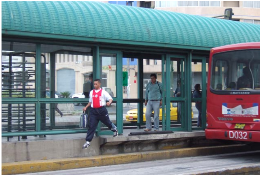
Fig. 11.60 Without sliding doorways, customers may evade fare payment and endanger their safety by entering and exiting through the platform doorway.
