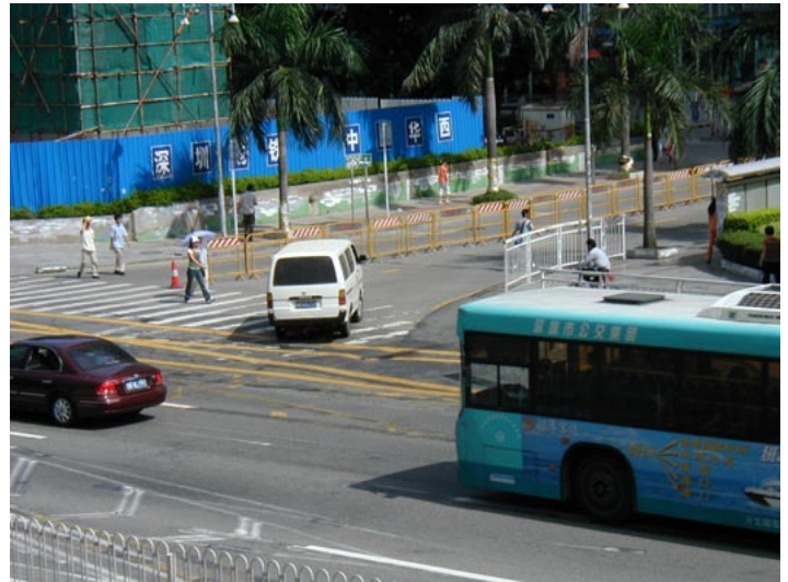
Fig. 13.30 A fence in the centre of the road keeps drivers from swinging wide during a turn in Shenzhen (China).
