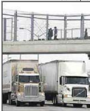
SAFETY: A pedestrian overpass was built at Huron Church and Girardot after a mother of three was killed there.
