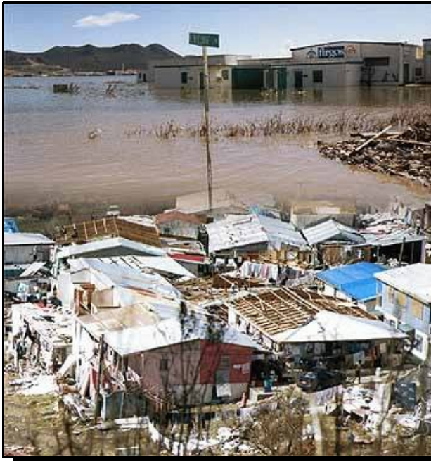
Wind and water damage caused by Lenny near the Salt Pond in Sint Maarten. Picture courtesy of Amigoe.
