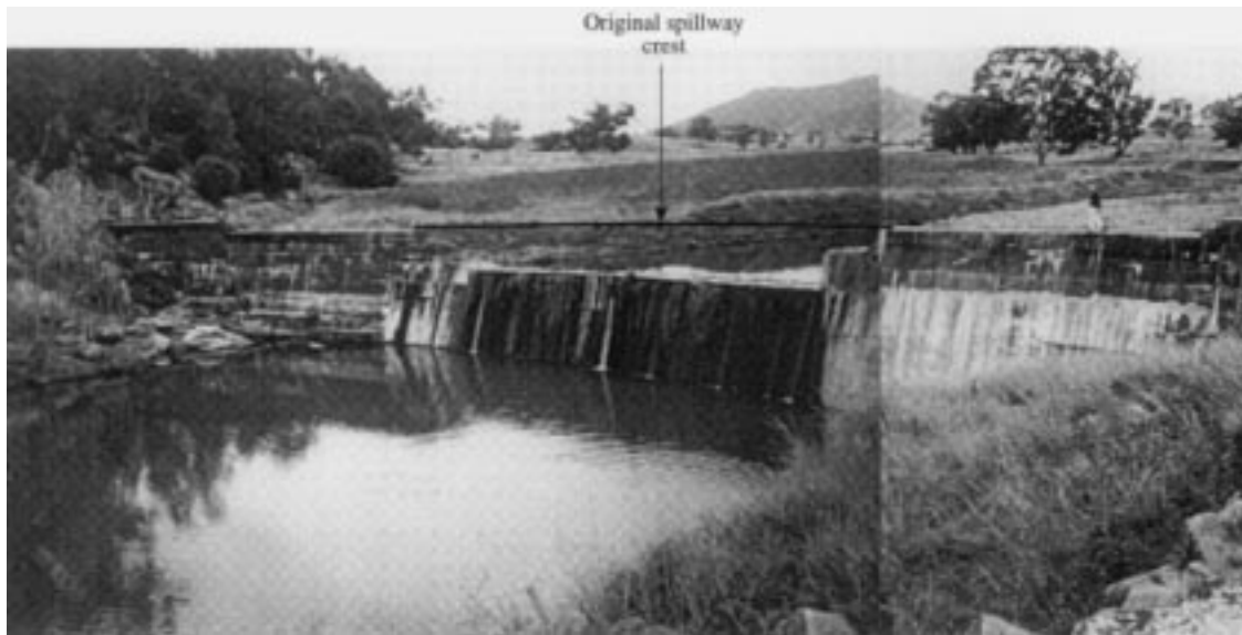
Fig. 4. The Gap Weir and its silted reservoir from a photograph taken on 13 June 1997 (by H. Chanson). The black line is the original spillway crest.
