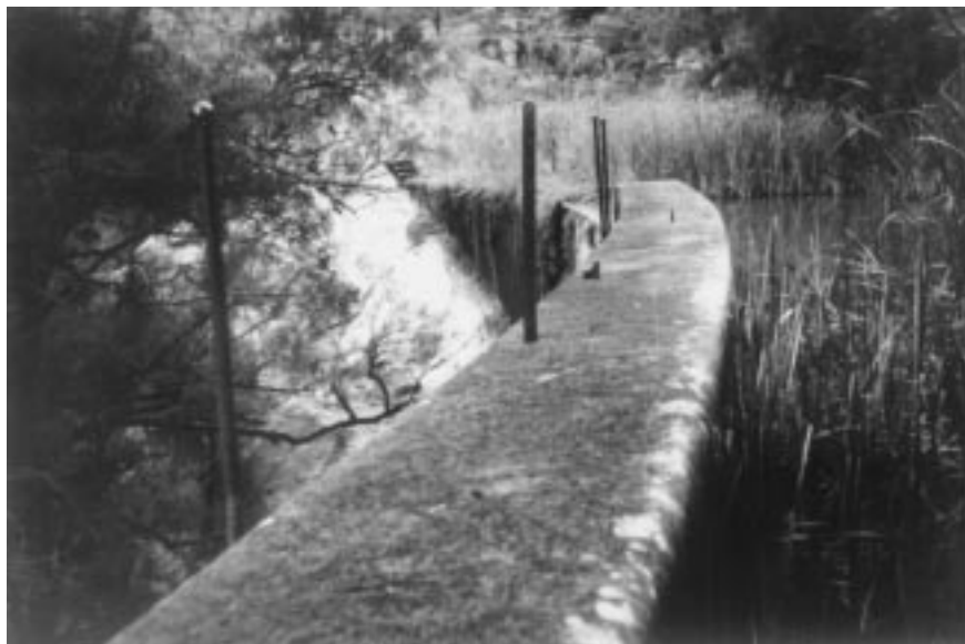
Fig. 3. Moore Creek Reservoir nowadays. Photographs taken on 14 June 1997 (by H. Chanson). (A) Downstream wall. The scour valve is visible just left of the tree. (B) Crest view, looking toward the right bank.
