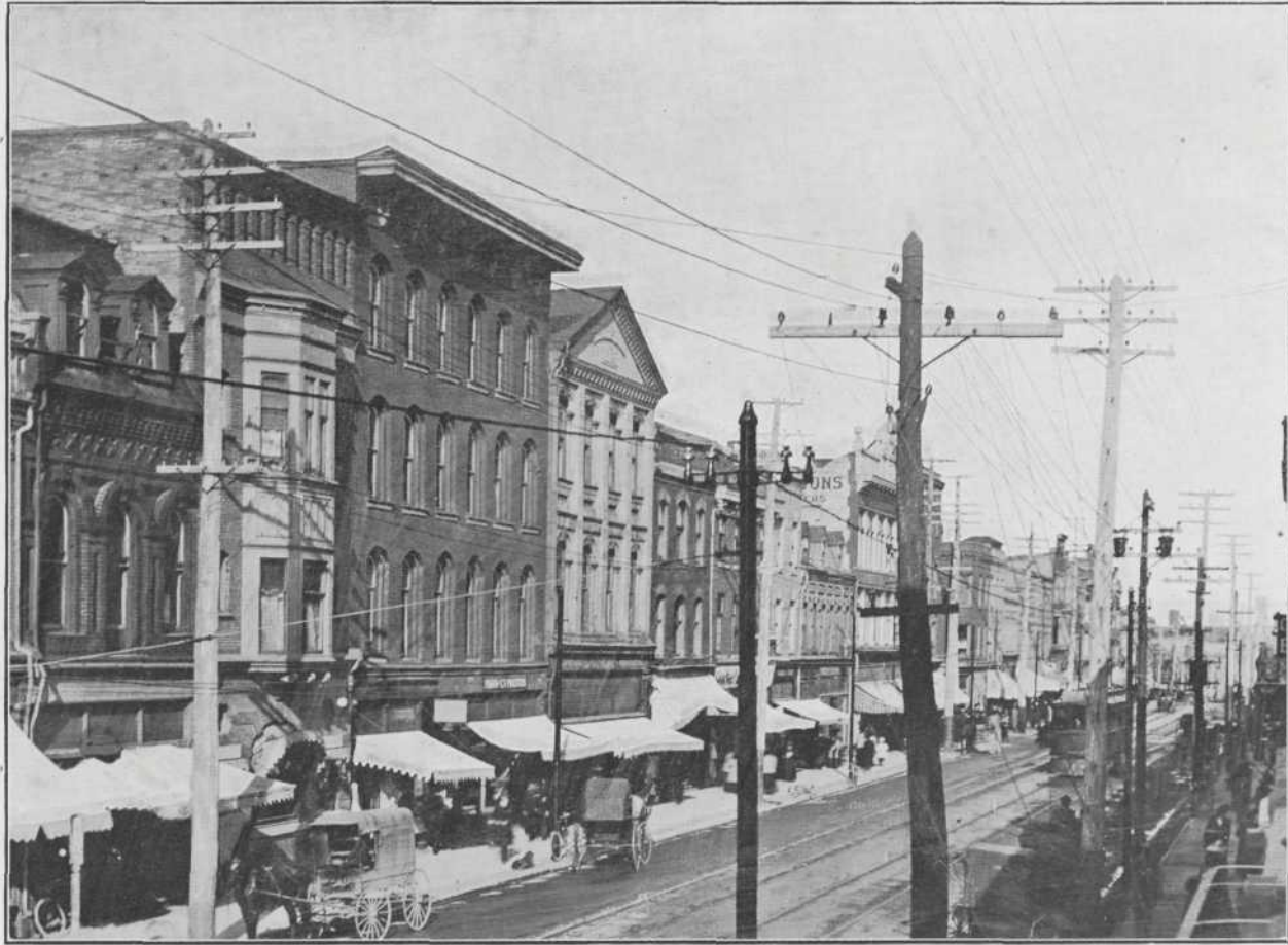
Colborne Street—One View looking East along the Main Business Street
