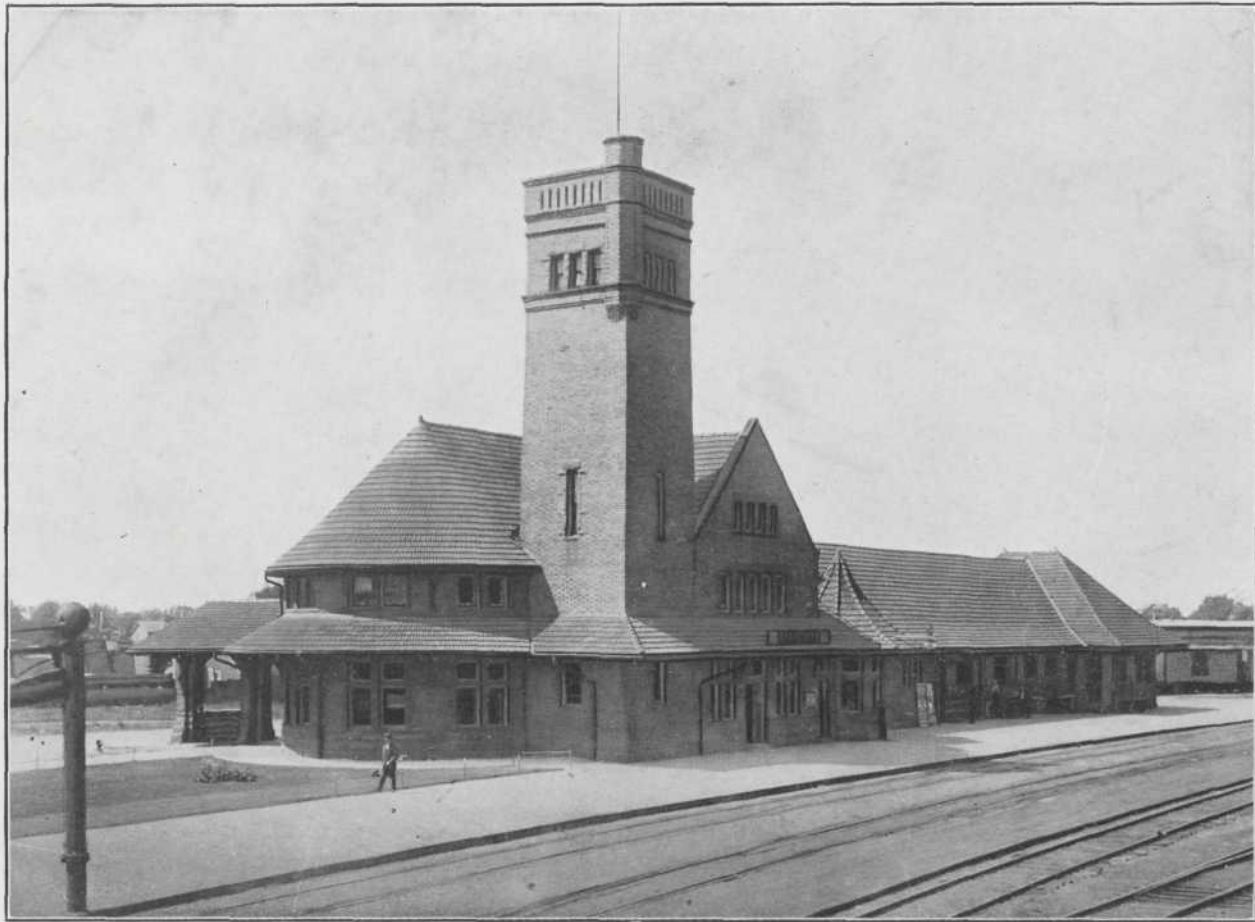
G. T. R. Station, Brantford, Canada— This is one of the most modern stations on the Grand Trunk System
