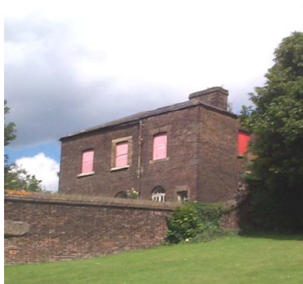
Kitchener barracks - Former Barrack Clerk's office, originally the Ordnance Store dated 1806.
