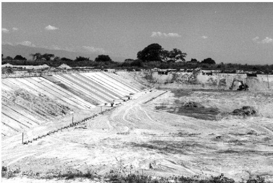
Construction of concrete liner on the side slopes of the primary treatment cells at the Los Guayos treatment plant.
