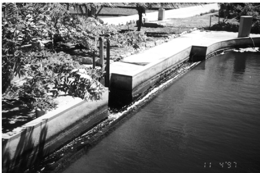
Effluent zone of the Juangriego basin operating in a decant mode.
