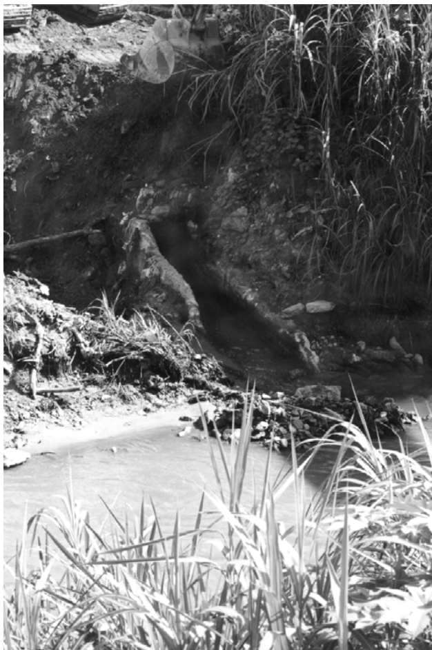
A raw sewage outfall into the Cabriales River. The Valencia sewage treatment project will intercept sewage from this discharge and many like it and convey it to the new Mariposa treatment plant.
