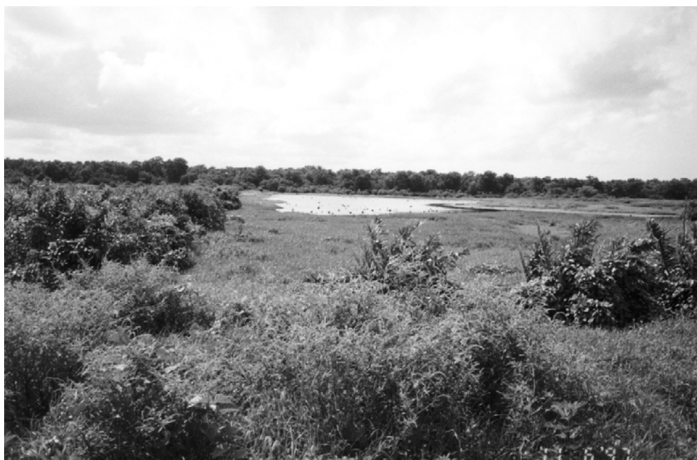
Lagoons at the Beetham Treatment Works are largely covered over with vegetation.
