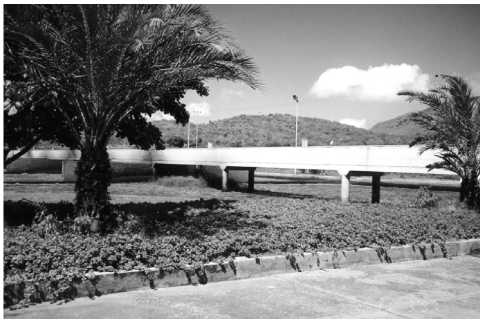
Aeration tanks at the Dos Cerritos treatment plant.
