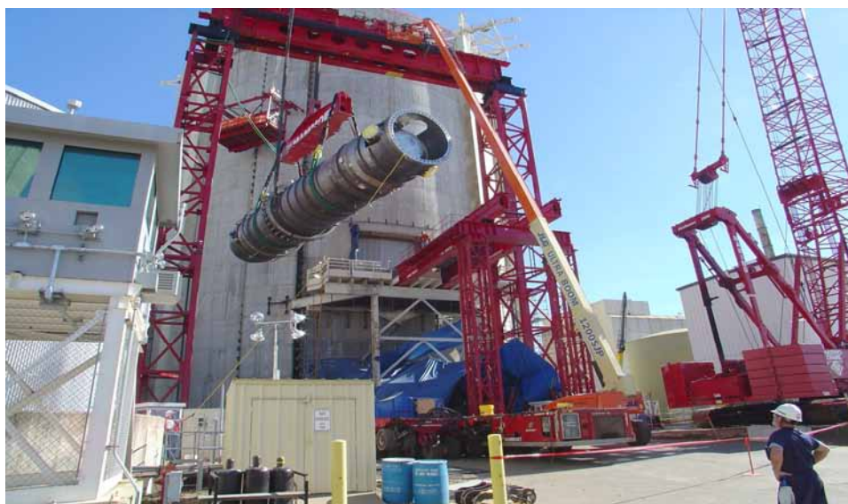
FIG. 21. SG rigging outside containment.
