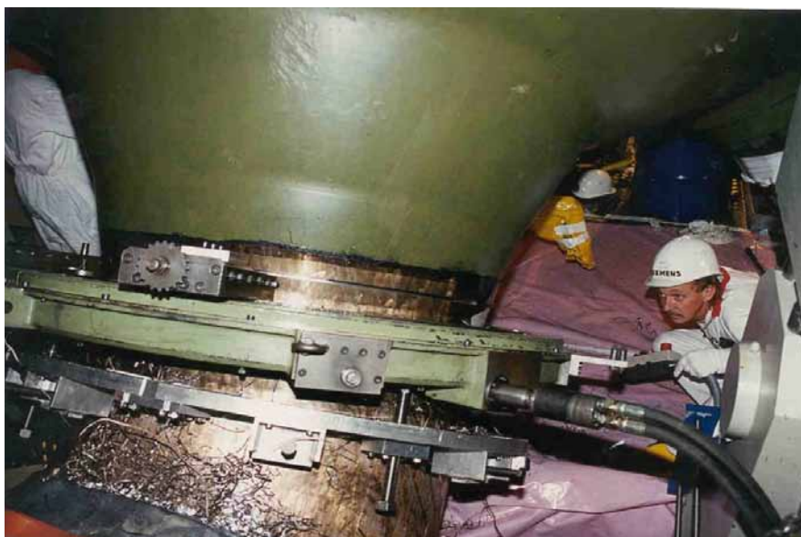
FIG. 16. Pre-cutting of the reactor coolant piping.
