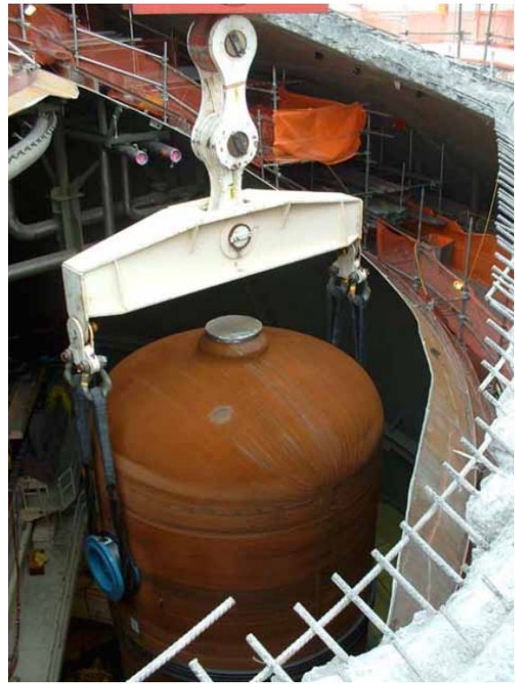
Fig. 24. Rigging SGR into containment building.
