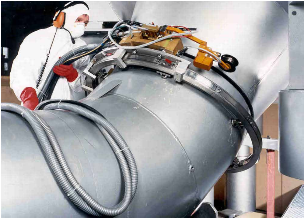
FIG. 13. Narrow gap welding equipment installed at the mock-up.
