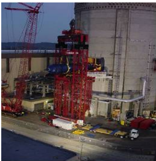
FIGs 26–29. Containment opening and handling/rigging.
