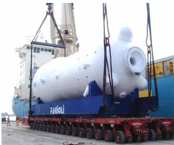
FIG. 19. Palo Verde Unit 2 SGR during transport.
