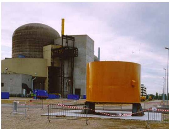
FIG. 62. Reactor vessel head on-site in its packaging before transportation.
