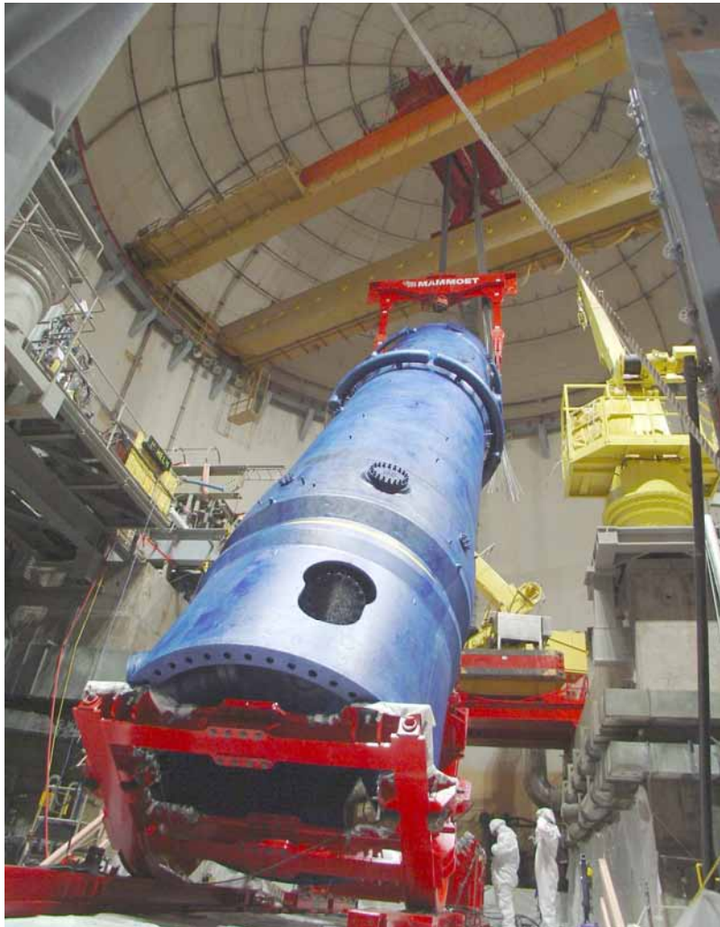
FIG. 22. SG rigging inside containment.
