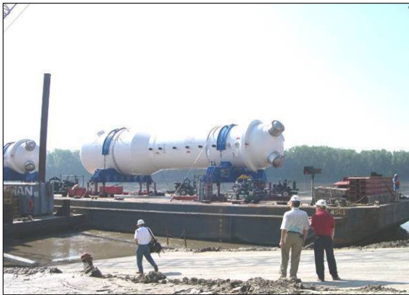
FIGs 30–33. Dock facilities at site for moving heavy components.
