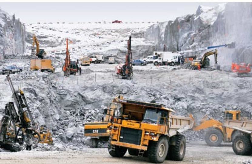
The Sarcelle powerhouse jobsite, in the Baie-James region.
