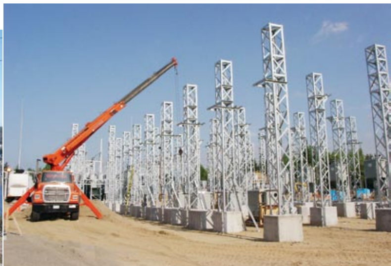
Construction of Saint-Lin substation (Laurentides).
