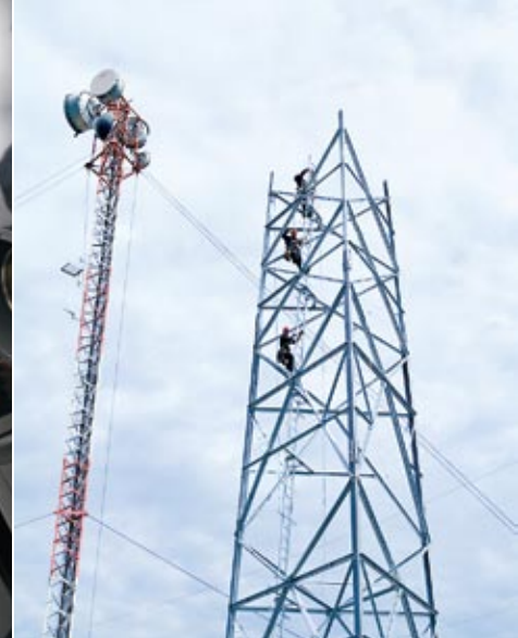
At Lévis substation, a new telecommunications tower stands next to a transmission tower under construction.
