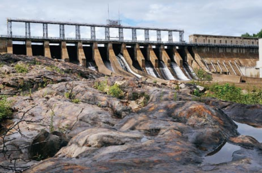
Mercier dam, in the Outaouais region.
