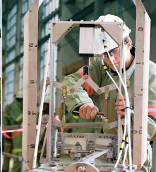
At Rivière-des-Prairies generating station, an engineer adjusts one of the components of the multipurpose submersible robot used to determine the condition of embedded parts.
