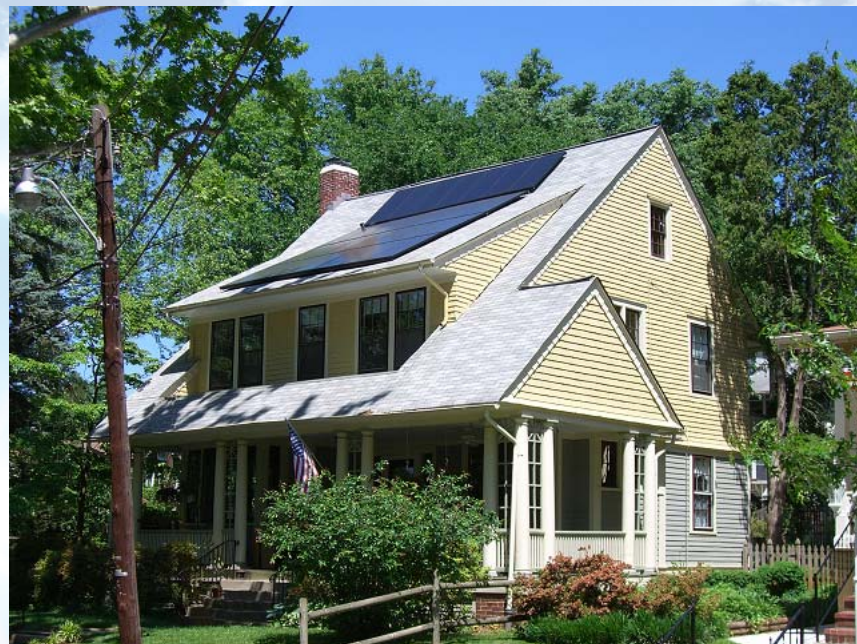
6-kW PV system provides 85 percent of this Washington, D.C. home's electricity. Courtesy: Standard Solar
