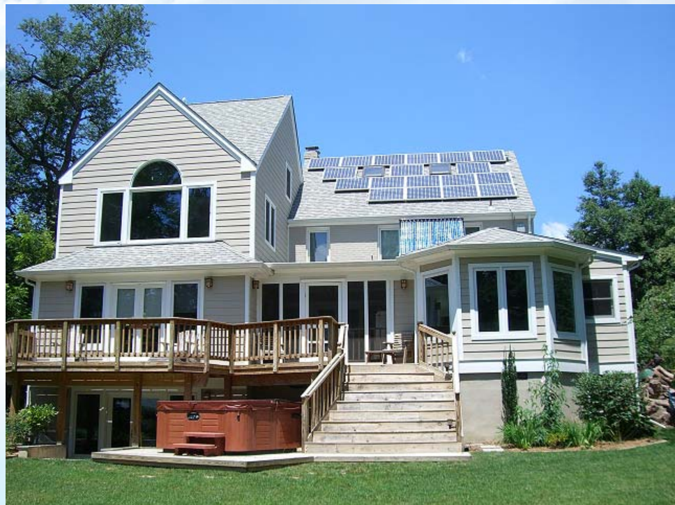
Home in Virginia with 80-gallon evacuated-tube solar water heater and 2.7-kW PV system. Courtesy: Standard Solar
