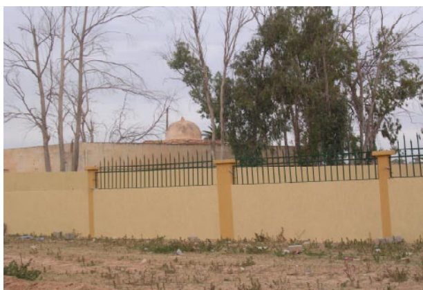
Figure 7 — A part of the new Azizia station fence
