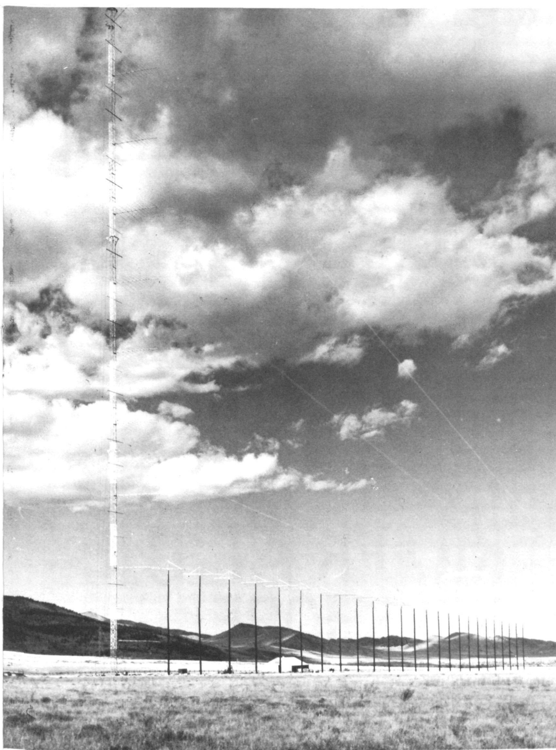
Antenna used to receive radio transmissions from the Ionospheric Beacon experiments on Satellites OGO-I and OGO-III.
