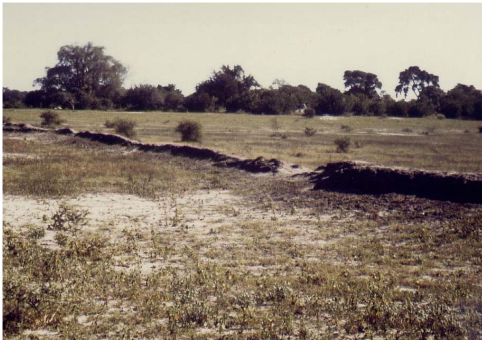
An old, abandoned, traditional bund made to retain the water for flood-recession cropping in the molapo
