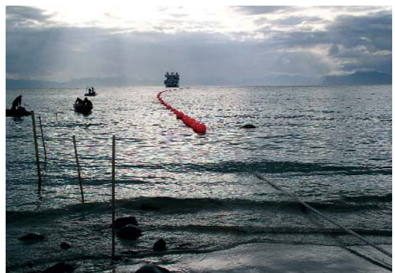
Figure 11 The cable ship installing the cable off the coast of Breivika
