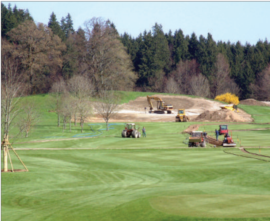
Construction on the 12th hole in April 2005.
