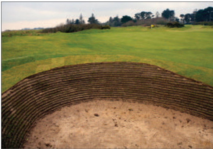
One of the new revetted bunkers currently under construction at Rosslare.
