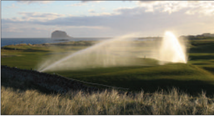
Toro's new Golf Decoder Controller system will make it easier for golf courses to control their watering.
