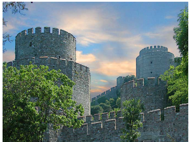
Fig. 7. Civilisation goes more than 7000 years back in time in Istanbul. The project is facing a major challenge in obeying the efforts required to ensure that all buildings and structures are unaffected and assuring that finds are preserved.
