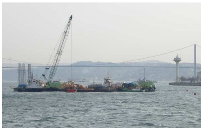
Fig. 3. Compaction grouting (at left end of barge).
