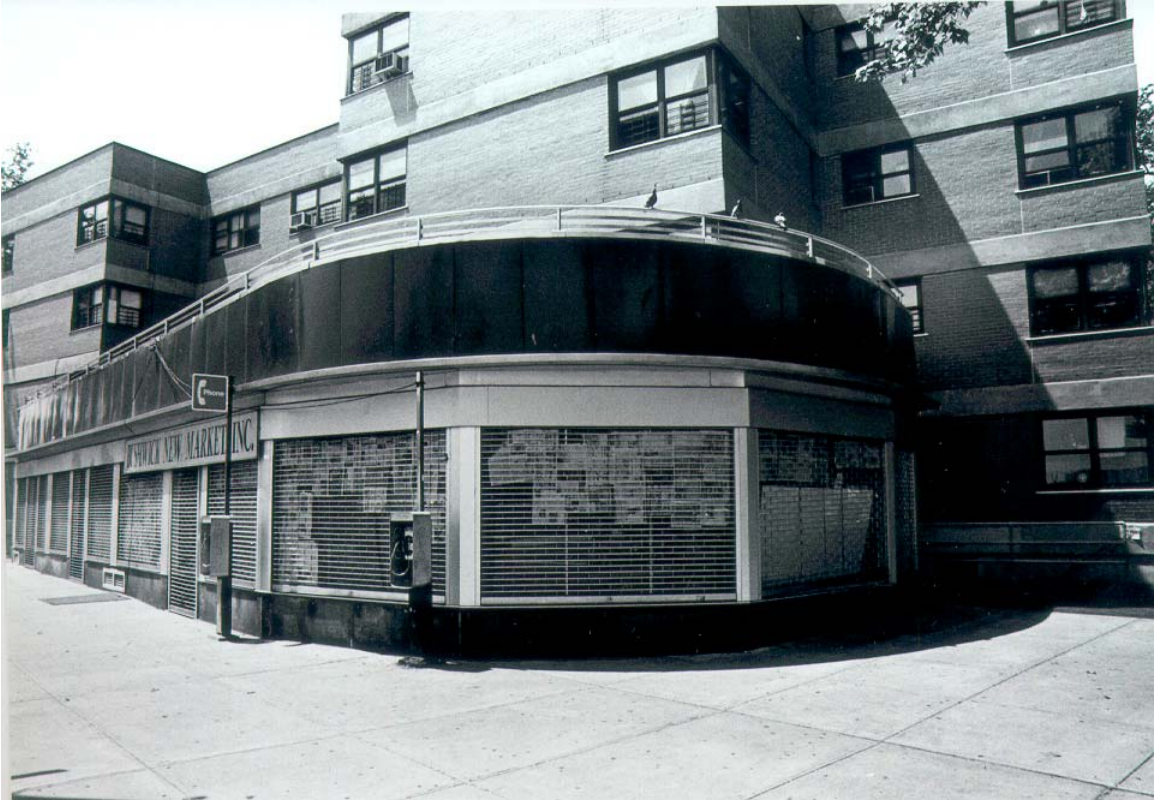
Williamsburg Houses Storefront at Bushwick Avenue and Stagg Walk
