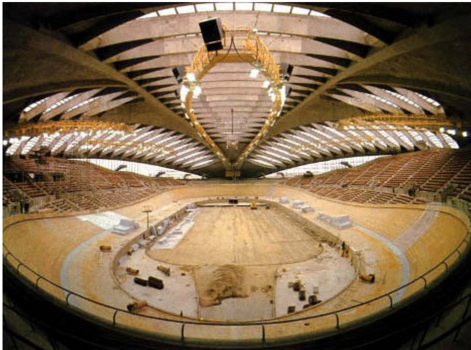
March, 1976: work on the Olympic Pool is proceeding on schedule.
