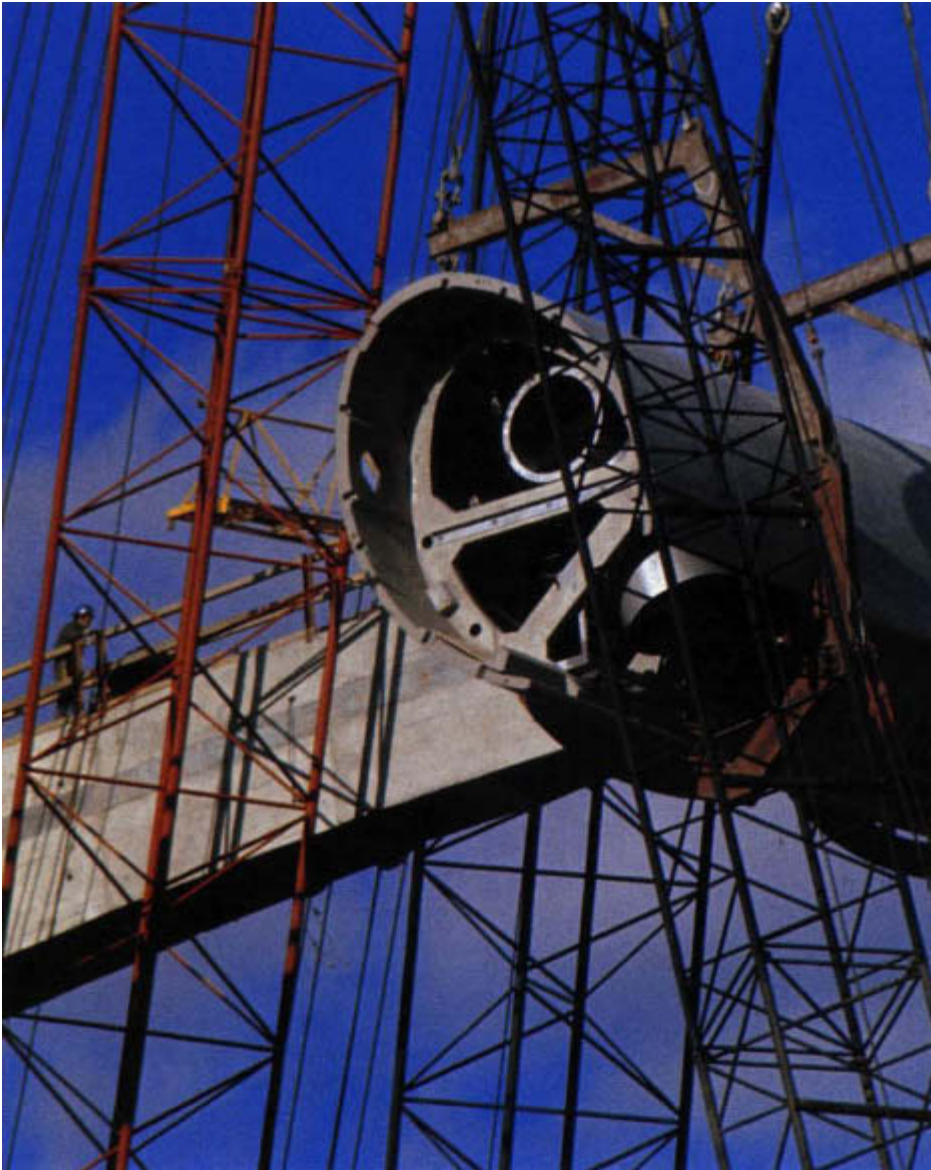
The Olympic Stadium on November 4, 1975: the first section of the technical ring is raised into place.
