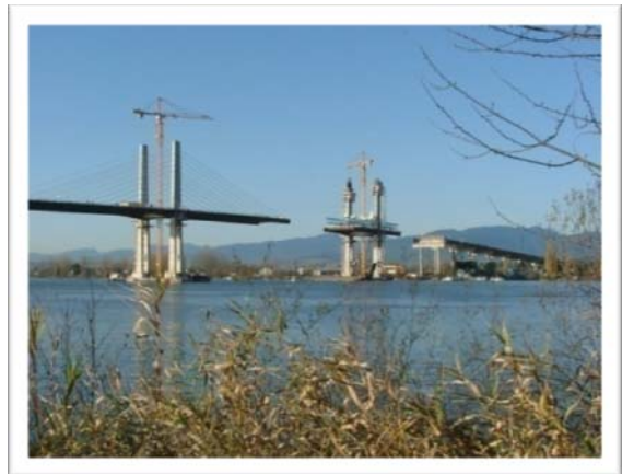
Courtesy of Golden Crossing Constructors. Bridge scheduled to open summer 2009
