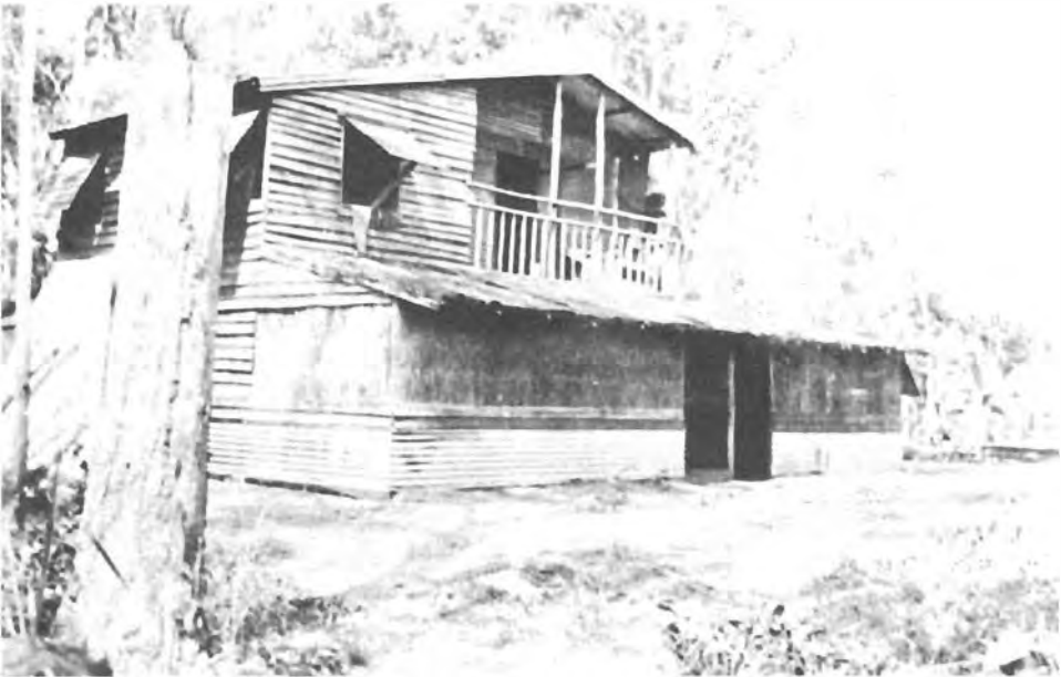
12. The mission house at Emerald River, Groote Eylandt before the March 1923 cyclone (H. L. Perriman collection N.T. Archives).
