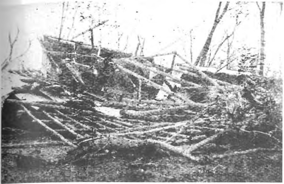
13. The mission house at Emerald River, a jumbled ruin after the 1923 cyclone. (H. L. Perriman collection N.T. Archives).
