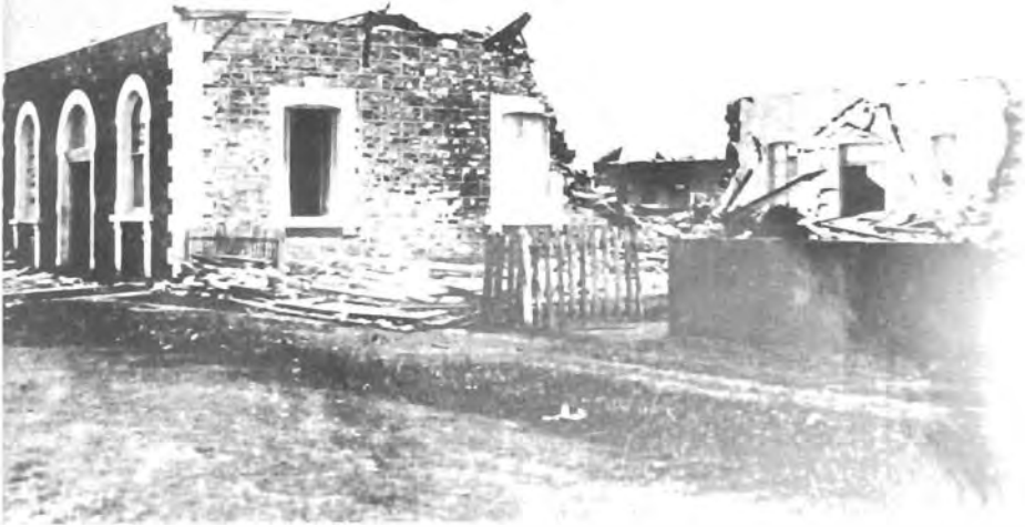
6. Damage to Mercantile building, Palmerston, January 1897. (South Australian Archives)
