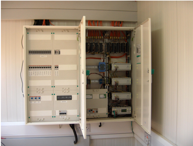
Fig. 4. Monitoring System at Photovoltaic Park. Cables from all outdoor sensors are terminated at the central datalogging system which stores and sends the data to a central database both at the Institute of Physical Electronics in Stuttgart and the University of Cyprus.
