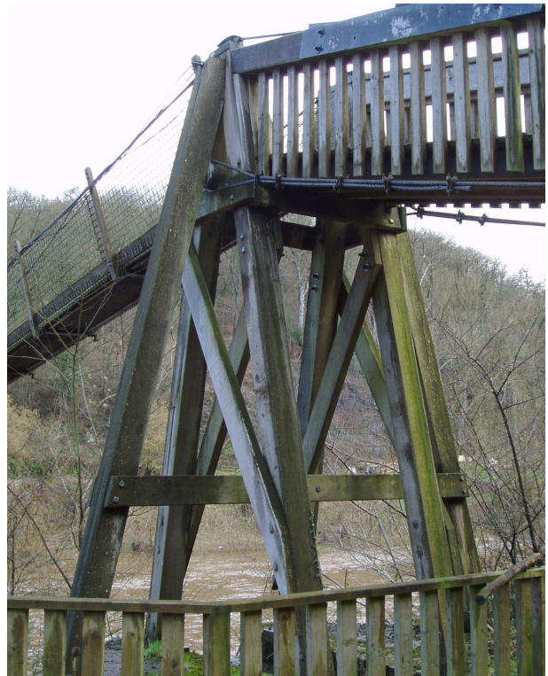
Figure 7: Tower construction, showing lateral bracing
