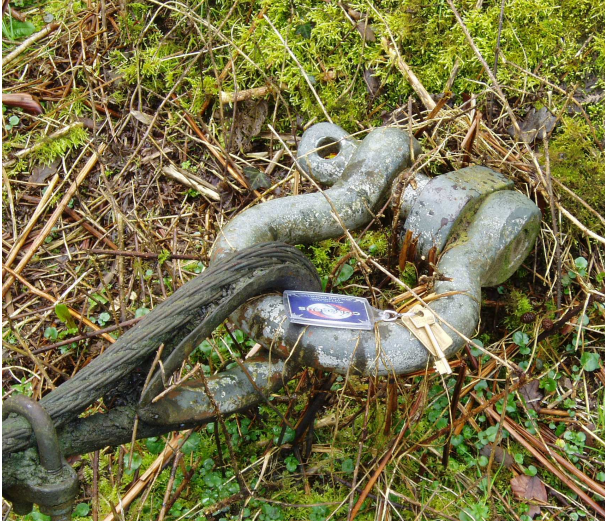
Figure 12: Attachment of main cable to abutment (key for scale).
