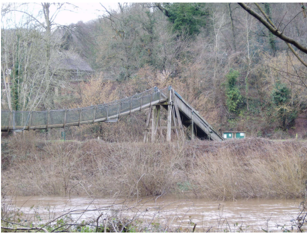
Figure 5: Biblins bridge in winter.
