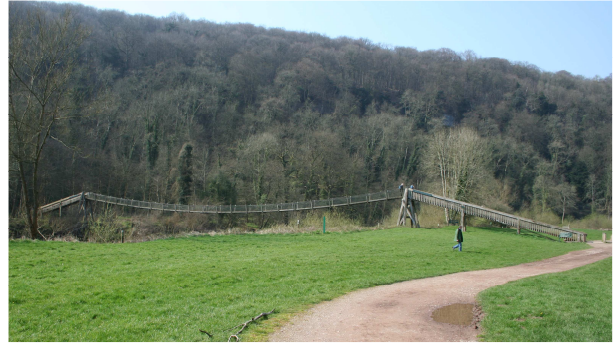
Figure 18: Biblins bridge from northern approach.
