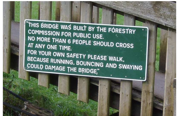
Figure 17: Sign on approach ramp to bridge.
