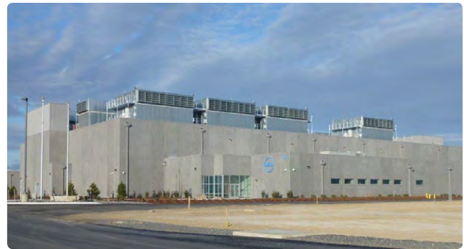
Dell's Western Technology Center in Quincy, Washington (U.S.), uses heat-wheel technology to reduce overall energy and water demands.
