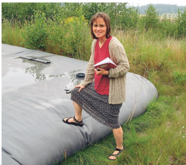
Figure 8. Urine storage tank made of a 150 m 3 plastic bladder at Lake Bornsjön near Stockholm, Sweden (photo commissioned by: E. v. Münch, 2007).
