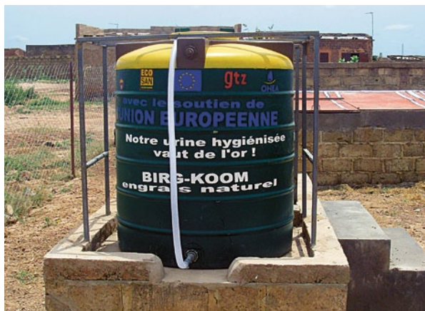
Figure 9. Plastic urine storage tank in Ouagadougou, Burkina Faso as part of the EU-funded project ECOSAN_UE led by CREPA (source: S. Rüd, 2008).
