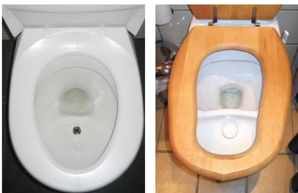
Figure 6. UD flush toilets. Left: Gustavsberg (in Meppel, the Netherlands); Right: Dubbletten (in Stockholm, Sweden); (sources: E. v. Münch, 2007).
