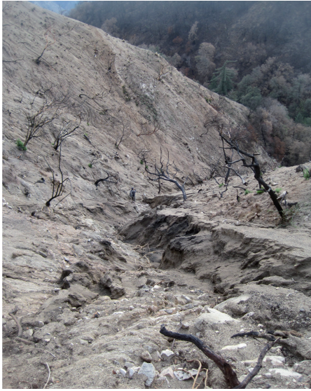
Fig. 7 - Photograph of channel erosion after the 18 Jan. 2010 storm (Storm 3). Geologist for scale in center of photo. Much of the channel bed in the foreground is bedrock
