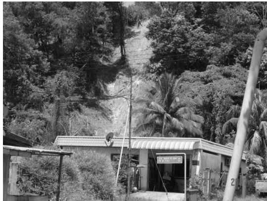
Figure 3. Landslide-prone area at Taman Po Hing housing estate.
