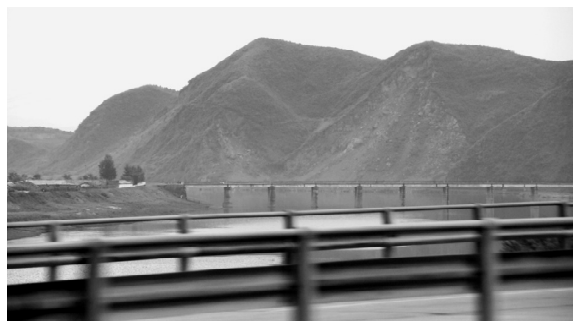
Fig. 4 Fault cliff landslides on triangular facet along Chonachon river fault system.
