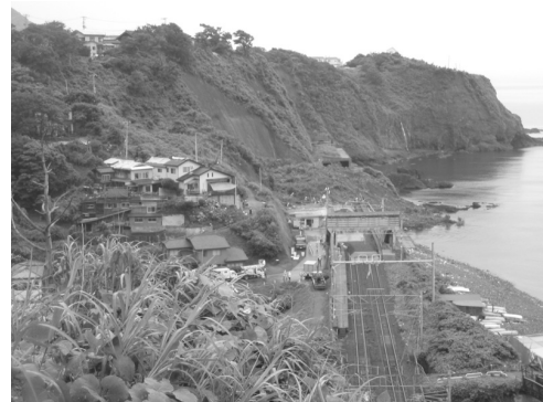
Fig. 1 A view of the Oumigawa landslide triggered by the 2007 Chuetsu Oki Earthquake, Niigata Prefecture, Japan
