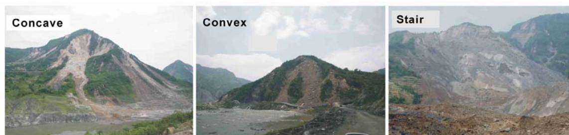
Fig.7 Typical sliding surface due to earthquake
