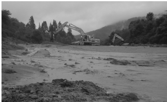
Fig. 4. The clean-up operation at the A9 north of Dunkeld.
