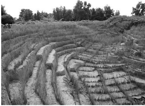
Fig. 5 This planting of Vetiver grass is about 3 months old. Vetiver grass has been shown to be an effective means of stabilizing slopes in many areas of the world and it is low-cost and relatively easy to apply.
