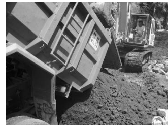
Fig. 9 Backfilling process
