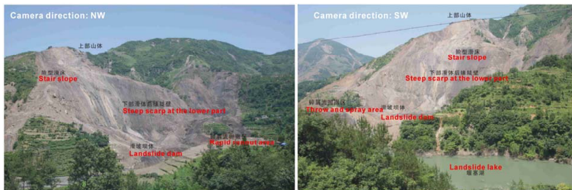
Fig.9 Stair-shaped landslide at the Taihong Village, Beichuan (150 deaths)
