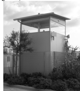
Fig. 6 Automatic Geodetic box in Marina Dorica
