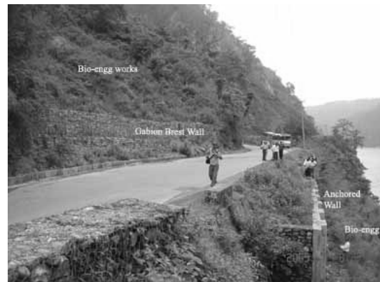
Fig 7: Photo of stabilized slope at Simaltal in 2008.
