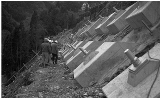
Fig. 8 Stabilisation works at Zentoku landslide on Shikoku Island, Japan
