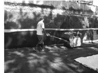
Fig. 10 Soil compaction
