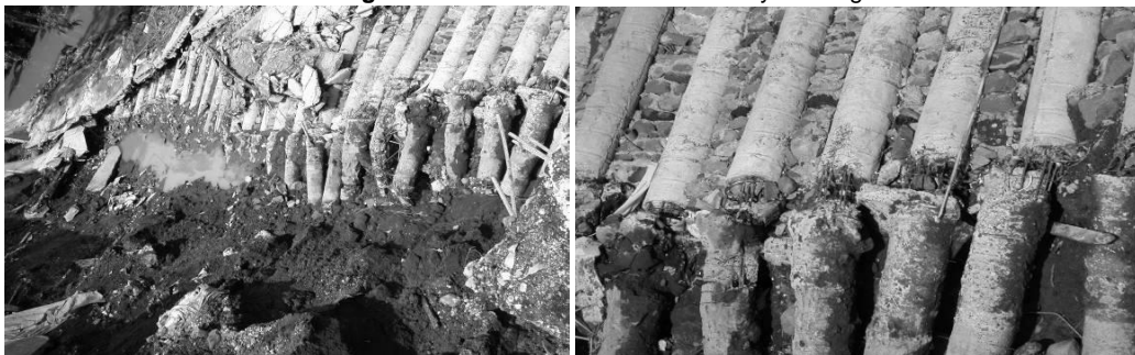
Fig. 2 The piles were broken and pulled out
