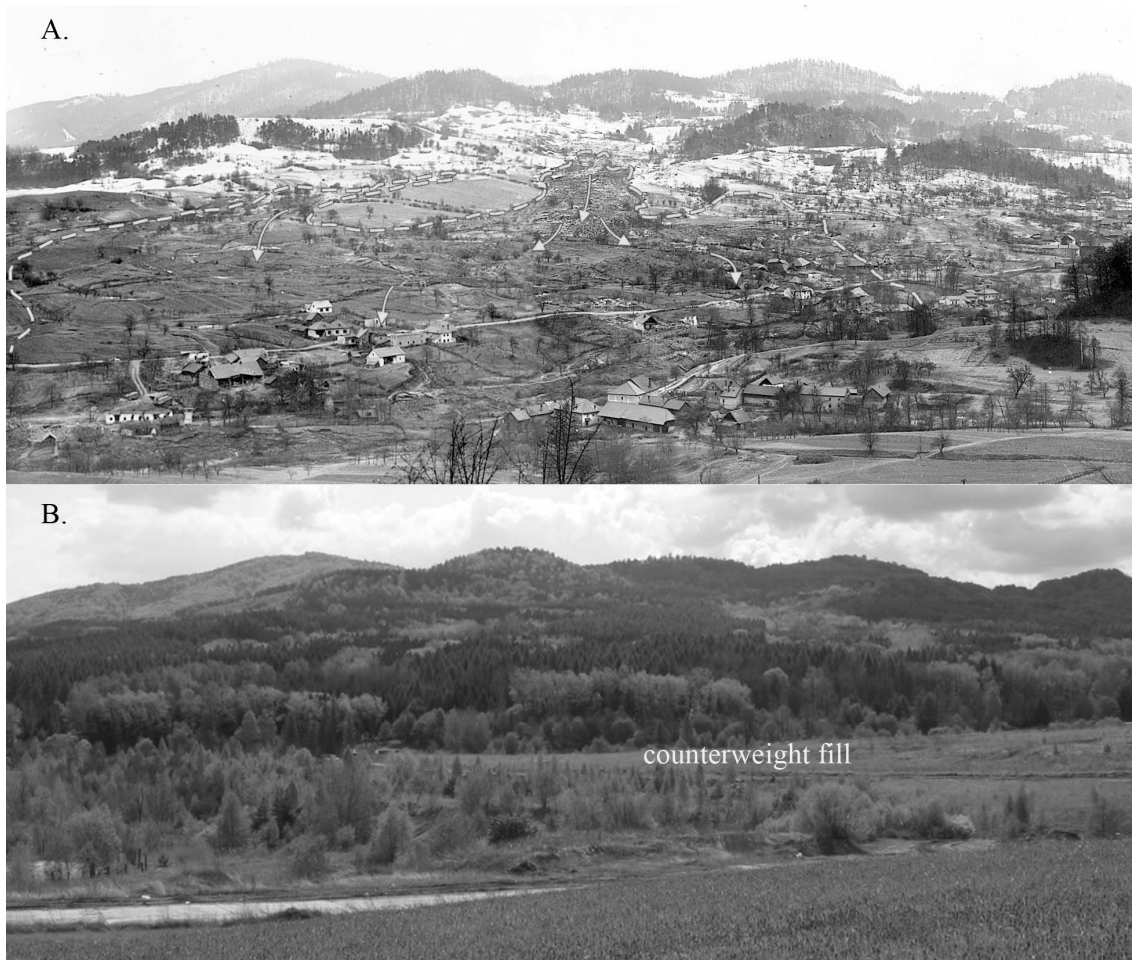
Fig. 4 Photos of landslide area in Handlova. A- lide in 1961 (photo by Nemcok and Malgot), B – present state of slope with counterweight fill at the toe (April 2008)
