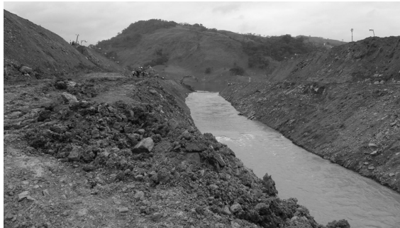
Fig. 6 Authorities opened a canal to avoid subsequent floods and a larger disaster
