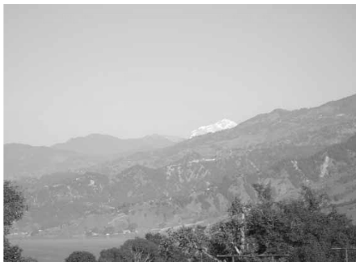
a. Slope failures in Phewa lake catchment (Kaski district)
