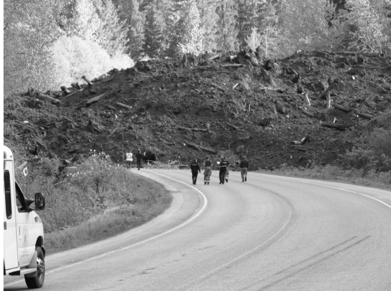
Fig. 6 Legate debris flow closed the Highway with the loss of two lives (Photo, G. Ross, BC MOTM 2007).
