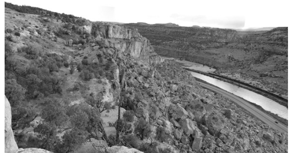
Fig. 6 DeBeque Canyon landslide showing Interstate 70 passing over the toe
