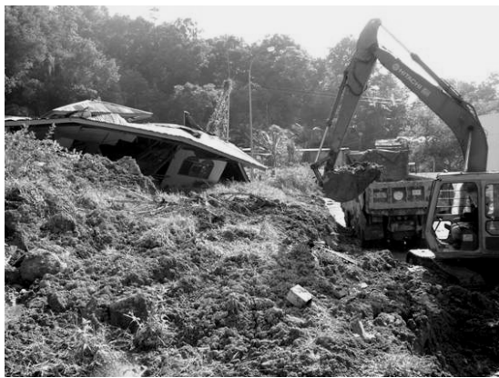
Figure 6. Houses buried during the Lok Bunuk 2006 landslide.
