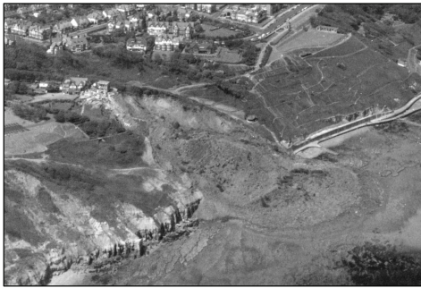
Figure 1 Holbeck Hall Landslide, Scarborough, 1993.
