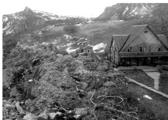
Fig.8 The front of a landslip has approached closely to "Visit-center" of Kronotsky Reserve, having destroyed only one of the electro-generator buildings.
