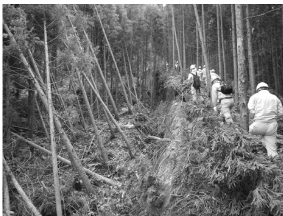
Fig.4-3 Photograph taken at the cliff
