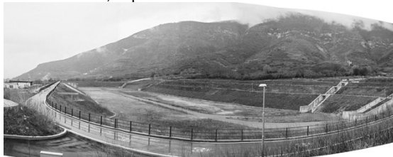
Fig. 9 Debris basin at Sarno in Italy
