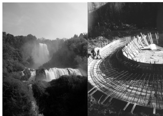
Fig. 7 Marmore Falls: remediation works
