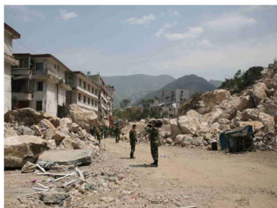
Fig.3 Destroyed road and houses due to huge rock falls
