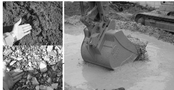
Fig. 3 Used fine and coarse material and its preparation
