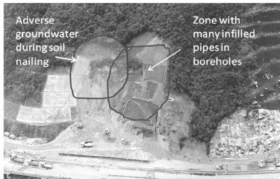
Fig. 8 Ching Cheung Road Landslide 1997
