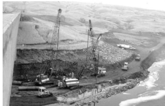
Fig. 2 Installation of stone columns around approach embankment fill area.
