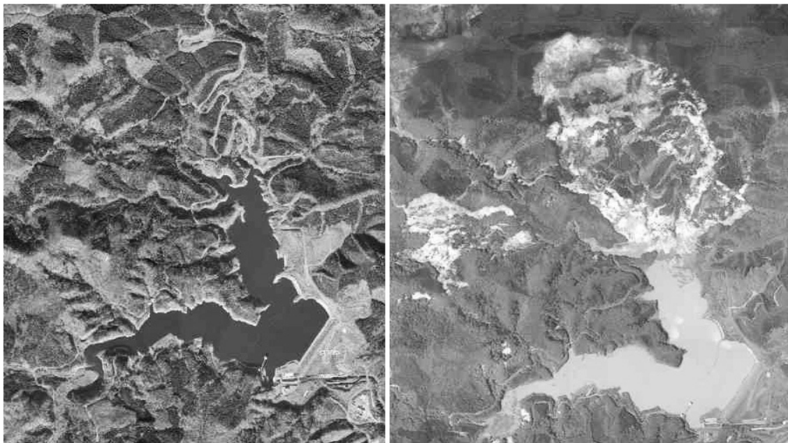
Fig.1 Before and after the huge landslide disaster that affected the Aratozawa Dam water reservoir
