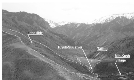
Fig. 3 The common view of the tailing and landslide in valley of river Tuyuk-Suu.
