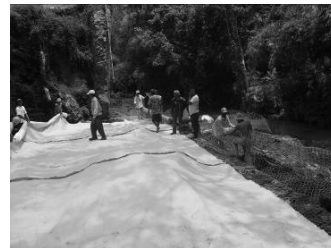
Fig. 8 Laying of composite geotextile
