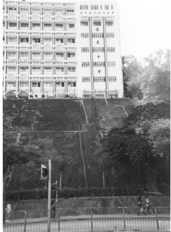
Fig. 7 A shotcrete slope in Kowloon, Hong Kong SAR
