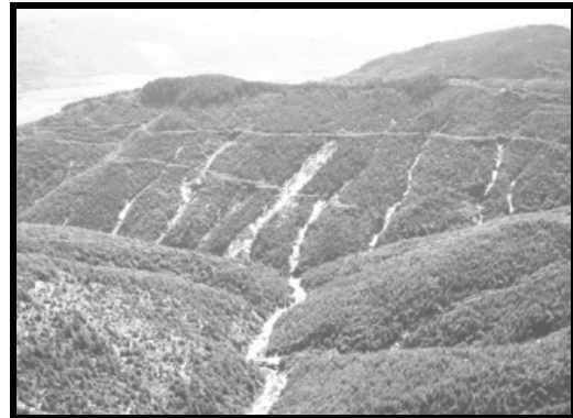
Figure 3. Road-induced debris flows in northwest Washington state, USA. The debris flows initiated in the colluvial hollows on the upper road were triggered by road runoff, and these triggered the failures at the road-stream crossings on the lower road. The road was built prior to the implementation of best management practices and large fill volumes were placed within colluvial hollow and inner gorge landforms.
