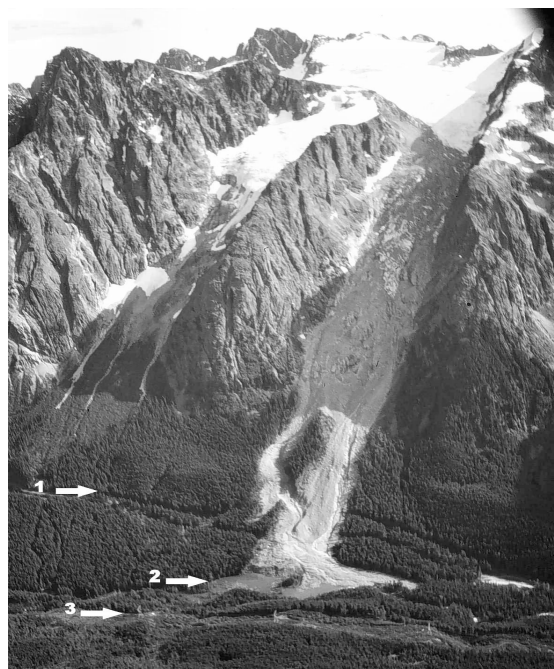
Fig. 4 Howson rock avalanche severed a natural gas pipeline. Arrows indicate: (1) the gas pipeline/access road; (2) a newly formed lake; and (3) the power transmission line.
