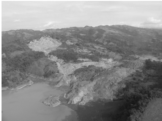
Fig. 3 Blocking of the river by the Grijalva landslide
