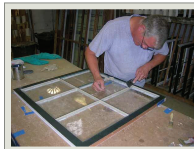
Woodcrafting team member Harold Hahn applies glazing putty to secure the glass panes in the newly manufactured wood window sash for Seminole Rest.
