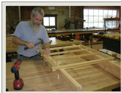
Woodcrafting team maintenance worker, Mark Stafford constructs new six-over-six double hung sash at the HPTC Jenkins Shop Facility.
