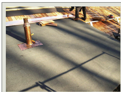
The HPTC crew was careful to "match in-kind" existing roof details such as the rolled roofing over the low sloped porch roofs.
