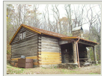
The "after" photo showing the completed FY2011 Pocosin Cabin project.
