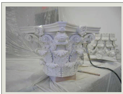
This photo shows the completed conserved column capital after painting.
