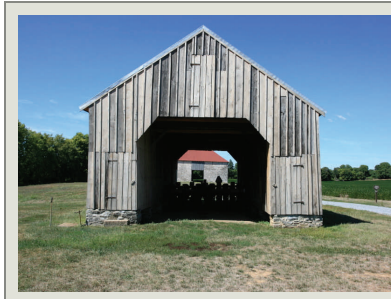
“Before” condition of the Corncrib/Wagon Shed which was constructed in the mid- or late nineteenth century and was used to store and dry corn and to shelter farm equipment.
