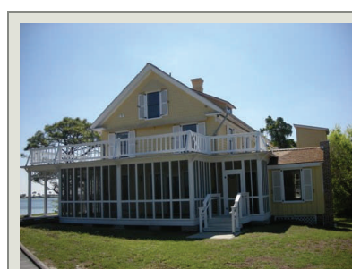
These two bottom photo's depict Seminole Rest "after" the HPTC had restored this Florida Coast home with historically appropriate windows, trim, roofing, and hardware.
