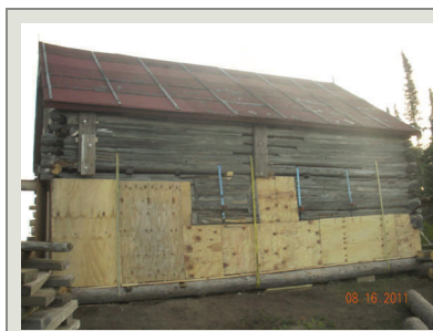
This photo shows an elevation of the Johns Hotel that has been temporarily stabilized using conventional lumber transported to the island. A second phase of work is required to finish this elevation.
