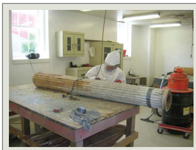
An interesting architectural feature of the larger HPTC Thomas House Interiors project was the conservation of two wood Corinthian Columns.
