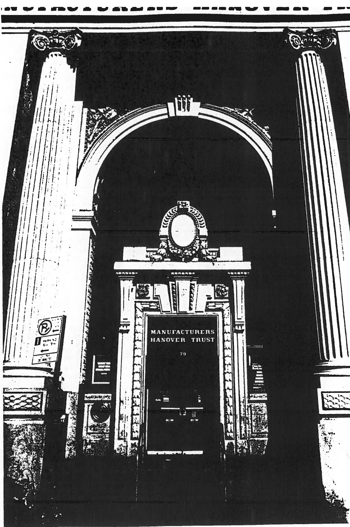
Manufacturers Hanover Bank Detail, Eighth Avenue facade, entrance
