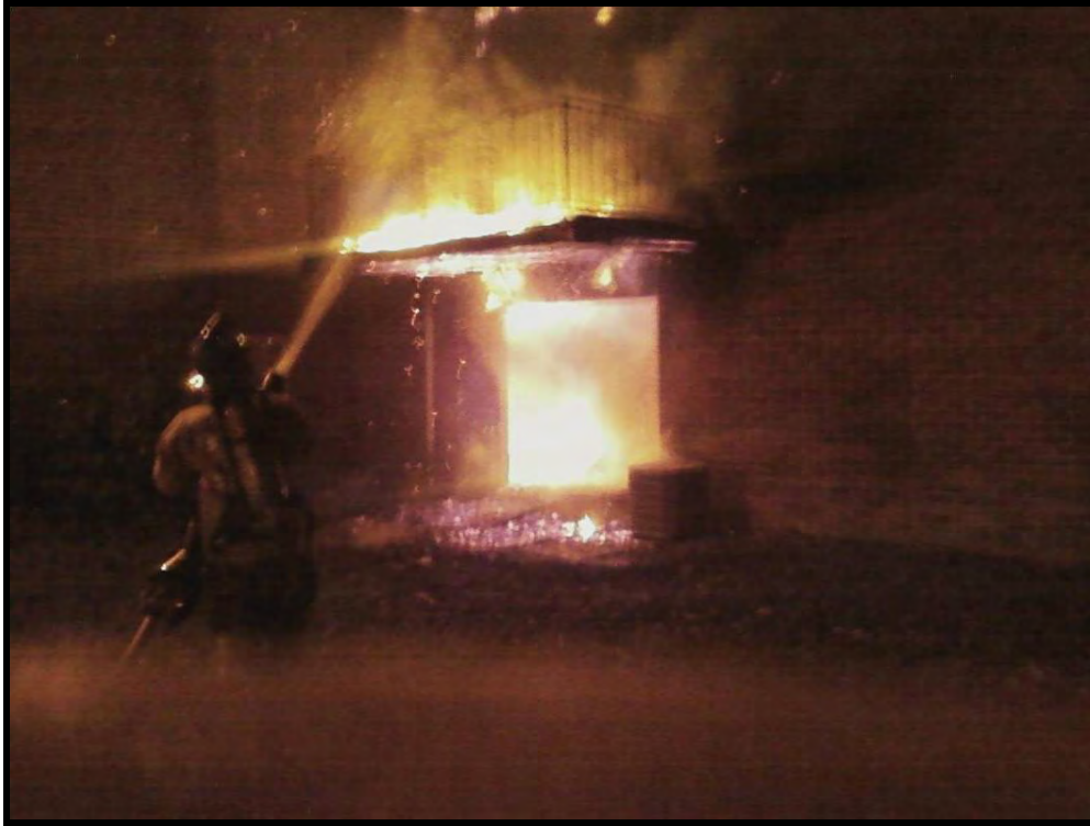
Figure 19. Photo of flame extension and suppression efforts at the rear of the structure. Flames caused the second level glass slider to fail and ignite plastic curtains in the doorway located at the top of the photo.
