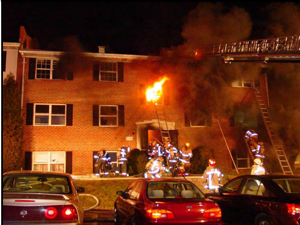
Figure 37. Photo showing flame extension through the stairwell to the third level. The stairwell window is broken by a ladder just after flames extend to the third floor. Evacuation tones are sounded just before this photo.
