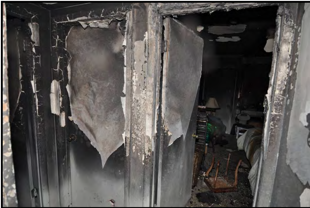
Figure 57. The left side hollow core door in this photo was shut by search crews after removing a victim from the living room to the bedroom. The living room reached flashover a short time later.
