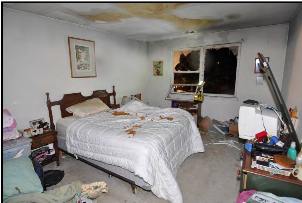
Figure 59. A second photo of same bedroom showing the VES window where the search crew entered and exited the apartment. Taking the time to shut the hollow core door blocked the ventilation flow path through the front window, thus isolating the crew and victim from the severe smoke and fire conditions in the hallway and living room.
