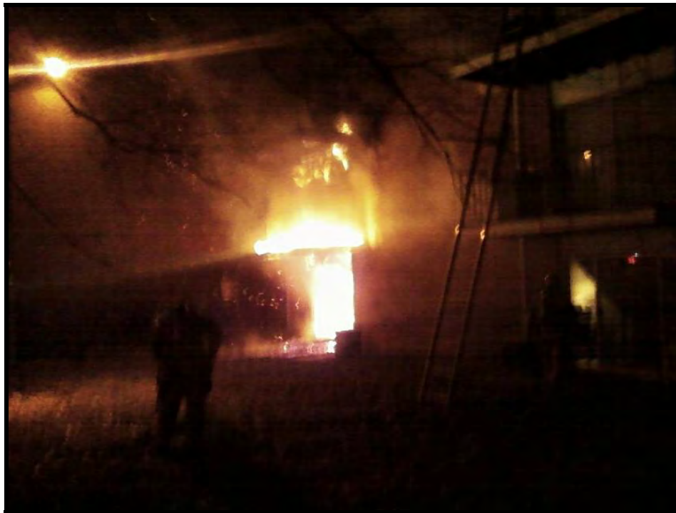
Figure 15. Photo from rear of flames in apartment T2 and extension to the balcony above. Note the relative minimal volume of smoke as the sliding door serves as the inlet for ventilation into the apartment. The smoke and heat is flowing in from the rear, through the apartment and up the stairs.
