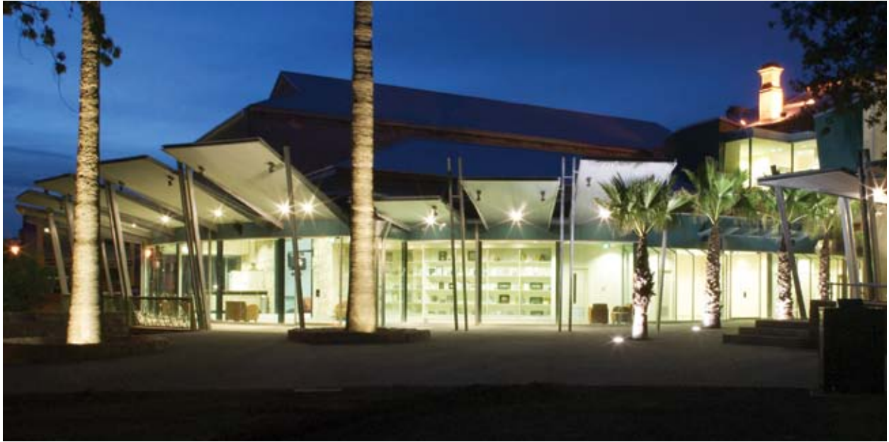
Award-winning redevelopment of Mount Gambier City Hall for new community uses
