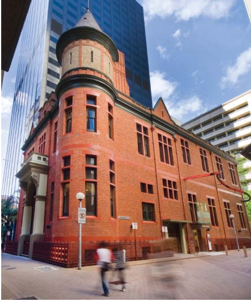
Former Adelaide Stock Exchange – The State Government will model best practice in the management of its own heritage assets*
