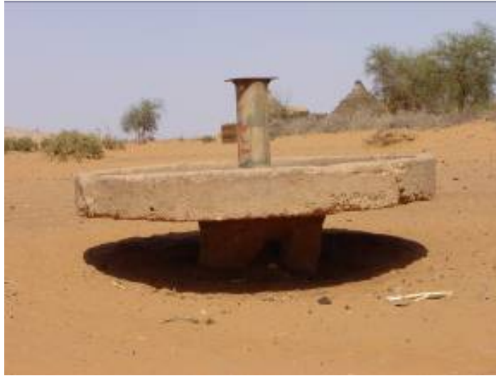
Figure 12: Inappropriate site selection
