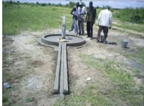
Figure 6: Platform and drainage apron construction for India Mark II hand pump
