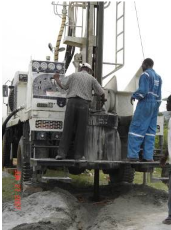
Figure 6: Borehole drilling in Juba, Southern Sudan
