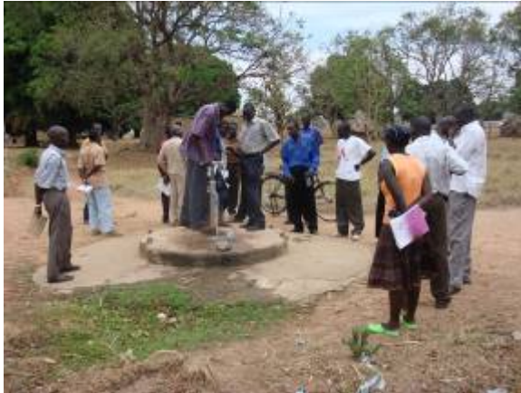
Figure 10: Direct action pump in use in Southern Sudan
